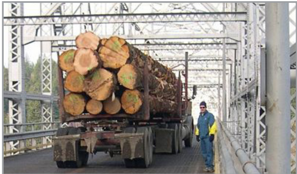
Pedestrian and logging truck share the bridge.
