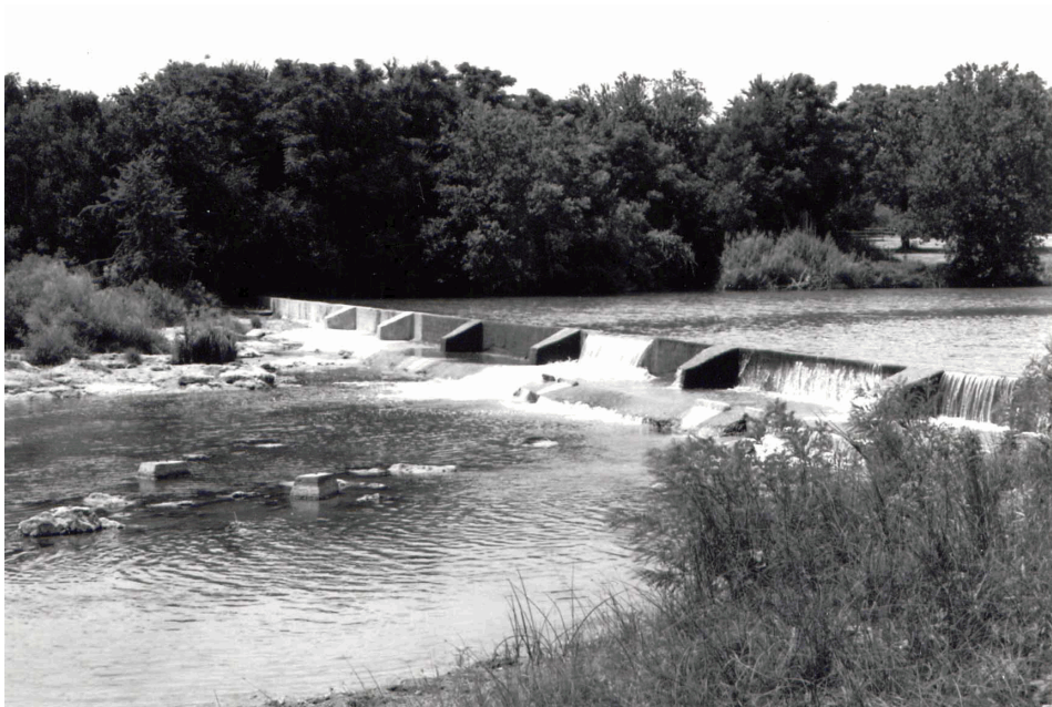
Jordan Dam constructed in 1944. Photo by E. Degutis, 1993.
