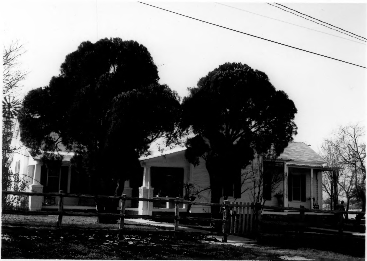
Front view of President Johnson's Boyhood Home in Johnson City, Texas. NPS photo taken 2/25/65 looking south.
