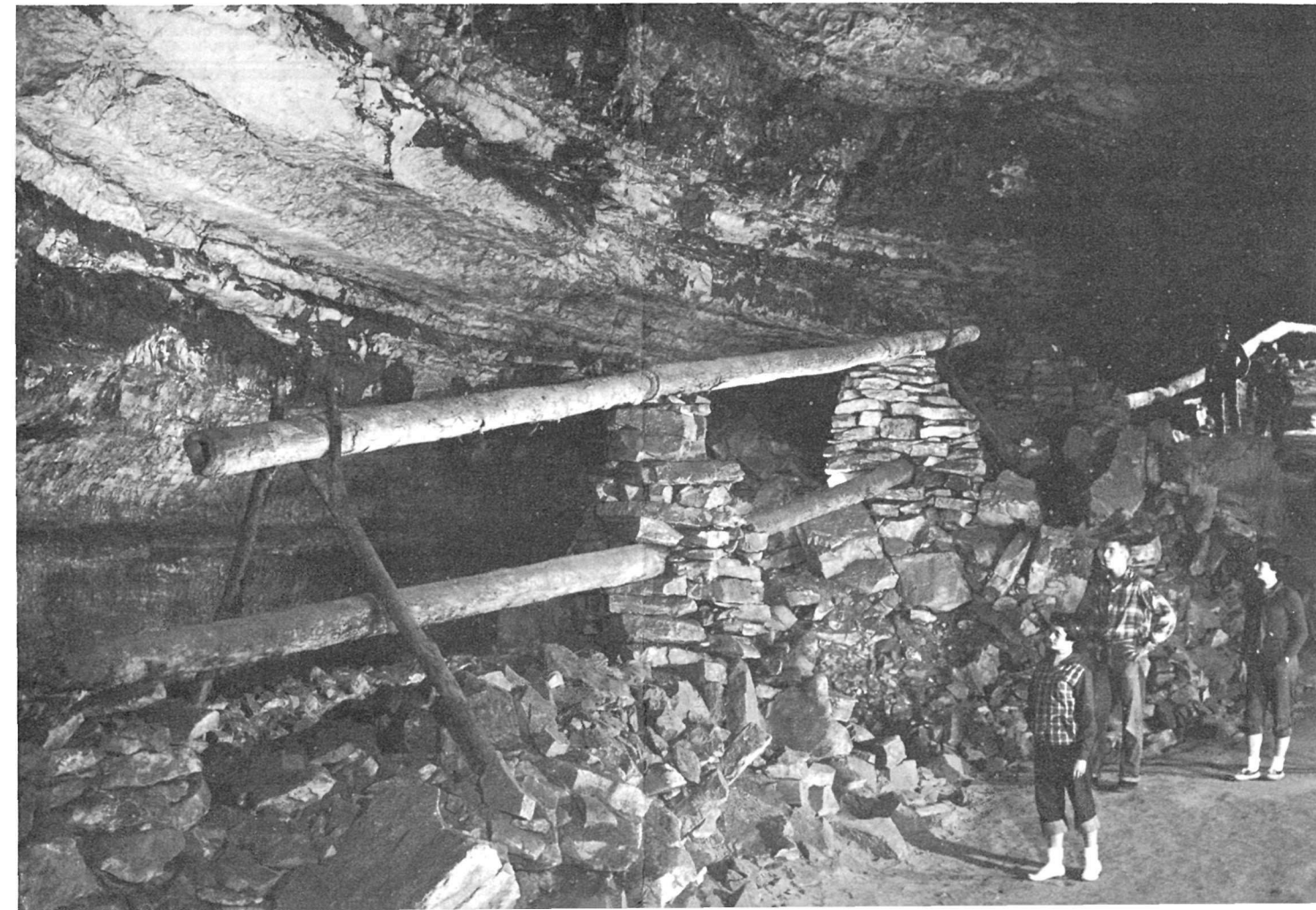
Wooden pipes used in saltpeter operations in War of 1812. Courtesy, National Park Concessions, Inc.; W. Ray Scott, photographer.
