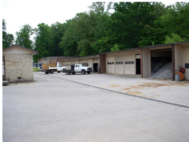
The park's maintenance yard showing the linear drain system that funnels runoff through a filtering system (NPS Photo by Dale Pate).
