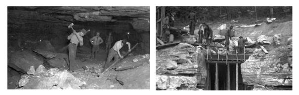
FIGURE 1-1. Two examples of cave modifications made by the Civilian Conservation Corps. Left is a photograph of trail building in the Historic Section, 1935; right, construction of the Frozen Niagara Entrance, 1938. (NPS images from Western Kentucky University, http://www.wku.edu/Library/nps/ccc).
