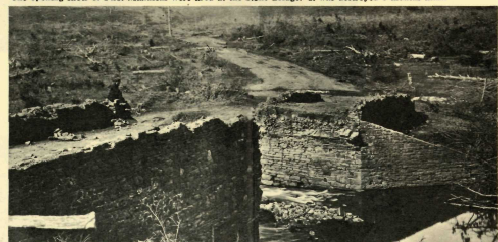
The opening shots of First Manassas were fired at the Stone Bridge. It was destroyed 8 months later.
