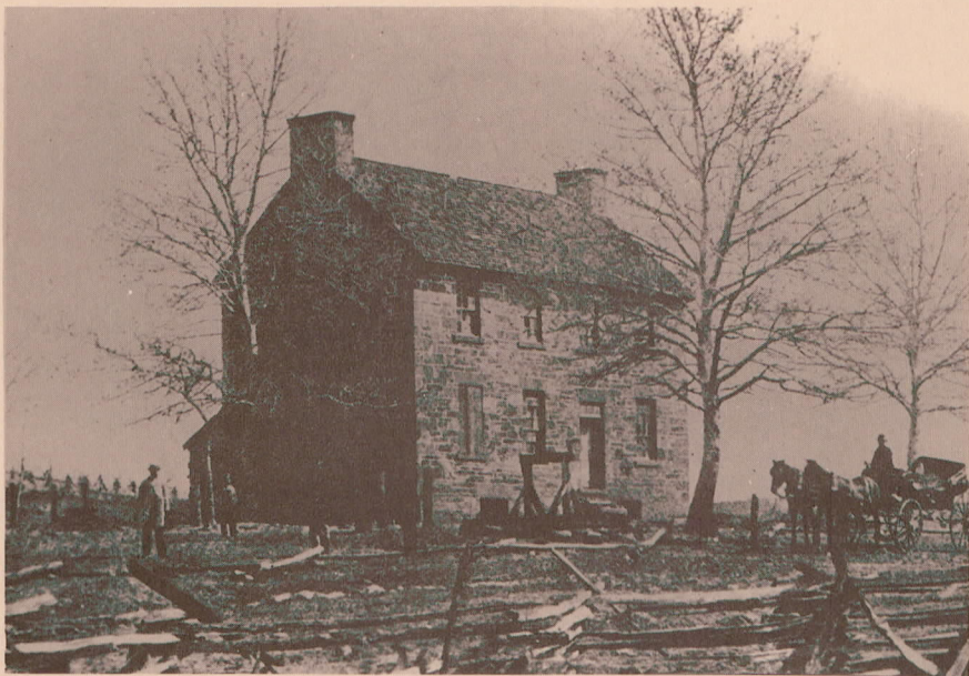
The effects of the First Battle of Manassas are evident in this photograph of the Stone House. Note the broken window panes, boarded-up window, and debris-strewn yard. Also of interest is the scaffolding on the roof; the Stone House was being reroofed when this photograph was taken in March, 1862.
