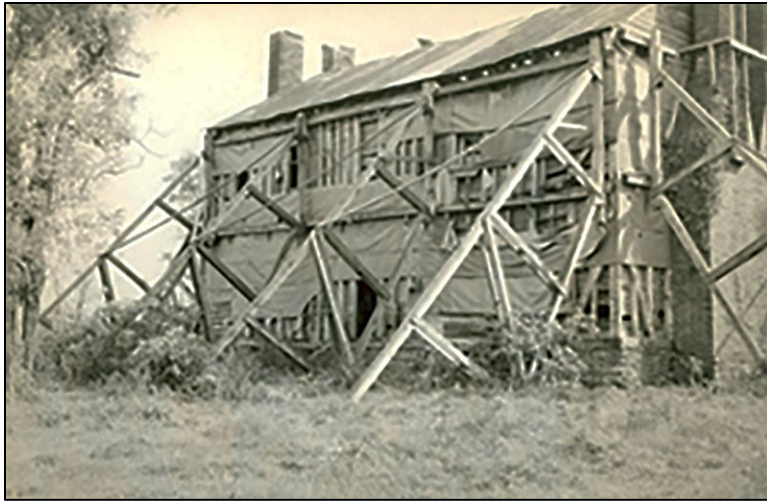
Fig. 24: Chinn House, weatherboards removed, tar paper installed, 1940, MANA Archives.
