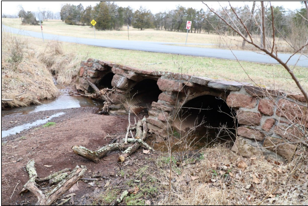
Fig. 31: South side of southern culvert over South Chinn Drive (NCR CLP 2023).
