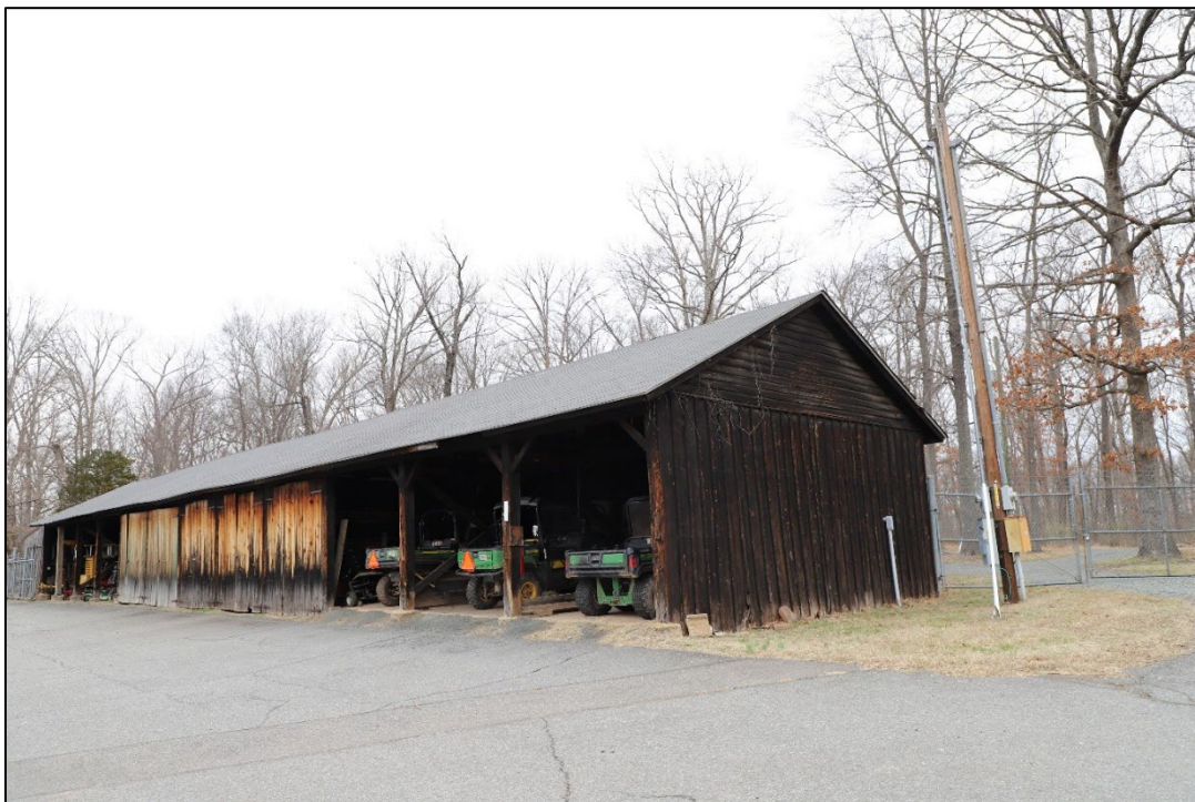
Fig. 27: Maintenance Storage Building east and south elevations, facing northwest (NCR CLP 2023).
