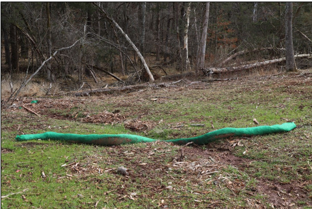
Fig. 15: Erosion control measures (NCR CLP 2023).
