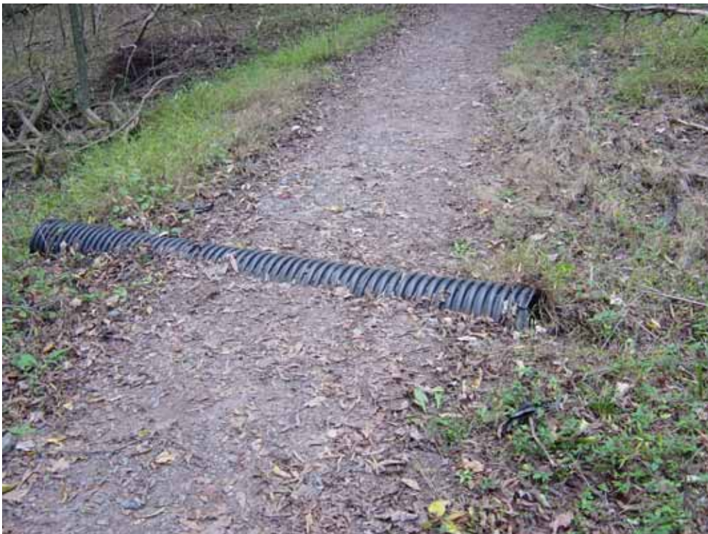
Figure 6. A temporary drain over a trail. Plastic piping is used to keep runoff from eroding trail and trail edges. Remedies such as this are temporary and often damaged by foot traffic. Photograph by Trista L. Thornberry-Ehrlich (Colorado State University).
