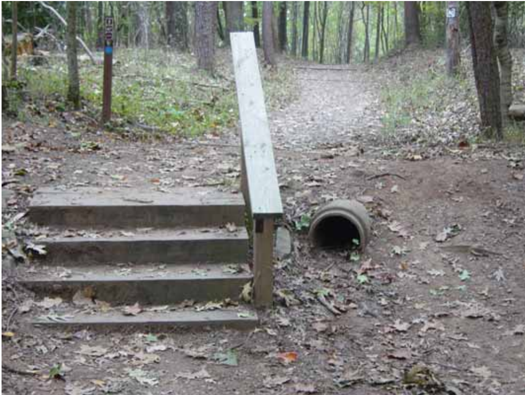
Figure 5. Erosion and widening of a popular trail (First Manassas Battlefield walking tour) at Manassas National Battlefield Park. Local seeps and springs create natural wet areas, which are especially prone to erosion. Stairs were built to concentrate foot traffic along this part of the trail, but the traffic has widened the trail beyond the stairs. Photograph by Trista L. Thornberry-Ehrlich (Colorado State University).
