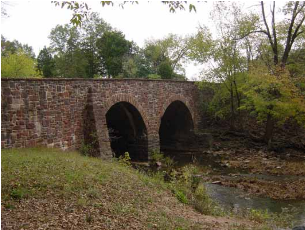
Figure 10. The old Stone Bridge over Bull Run. The bridge is located on an outcrop of Balls Bluff Siltstone. Because this siltstone is locally fractured there is the potential for instability of the bridge's foundation. Bridges were commonly situated in areas of exposed stone to provide a stable construction base. Photograph by Trista L. Thornberry-Ehrlich (Colorado State University).
