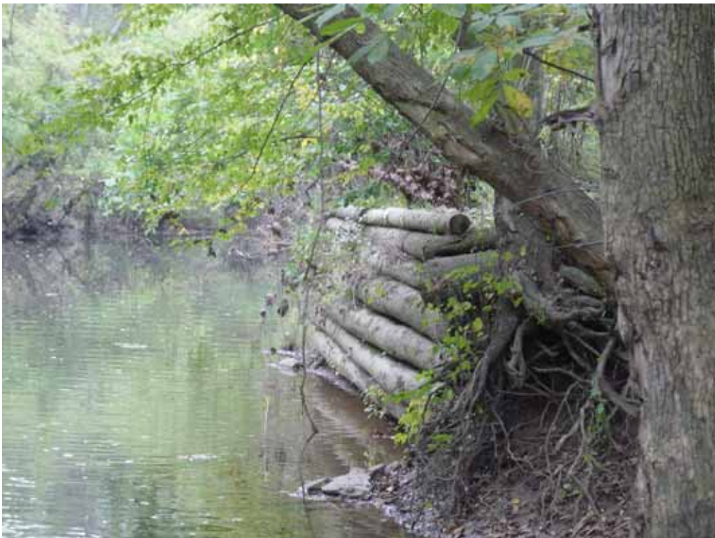
Figure 3. Buttressing along the banks of Bull Run. Structures such as this are placed to preserve a stream bank from erosion. One of the park's most traveled trails is atop this structure. Slopes along the banks of Bull Run can be high, accelerating erosion. Erosion has already exposed the tree roots (visible in lower right part of photograph). Photograph by Trista L. Thornberry-Ehrlich (Colorado State University).
