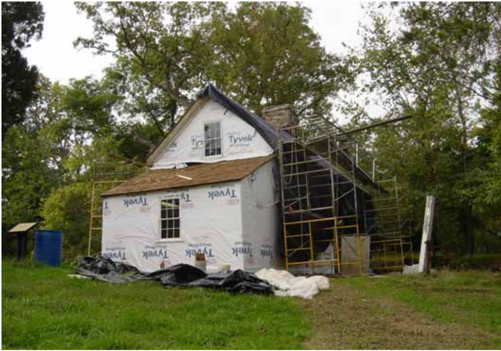
Figure 7. Restoration and preservation efforts at the Thornberry House, near Sudley Springs Ford in the northernmost corner of the park. The building was used as a residence, field hospital, and post office during its long history dating back to before the Civil War. Efforts include stabilizing the foundation and restoring slopes around the structure. Photograph by Trista L. Thornberry-Ehrlich (Colorado State University).
