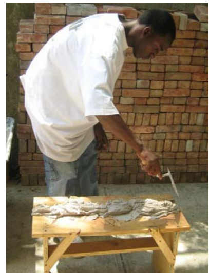
At DC student prepares mortar.
