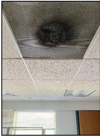
Figure 3: Suspected Mold on Ceiling of a Dispatch Center Office (Sept. 27, 2021)
