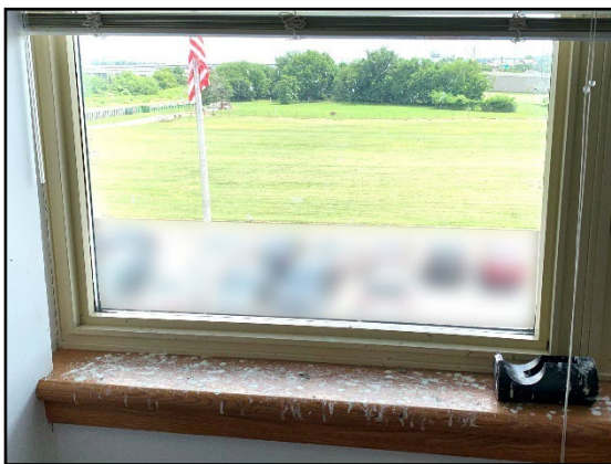
Figure 1: Bird Droppings in a Dispatch Center Office (July 1, 2021)*
