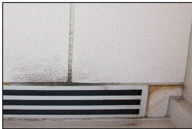
Figure 2: Suspected Mold on Ceiling of Dispatch Center (Sept. 27, 2021)
