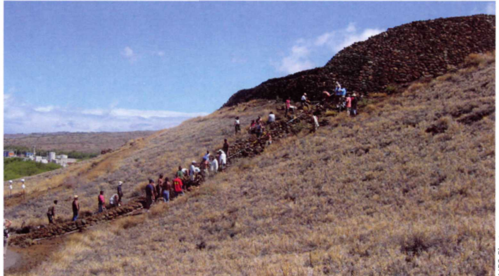
Crews rebuild the wall at Pu'ukohola Heiau NHS, which was damaged by an earthquake in 2006
