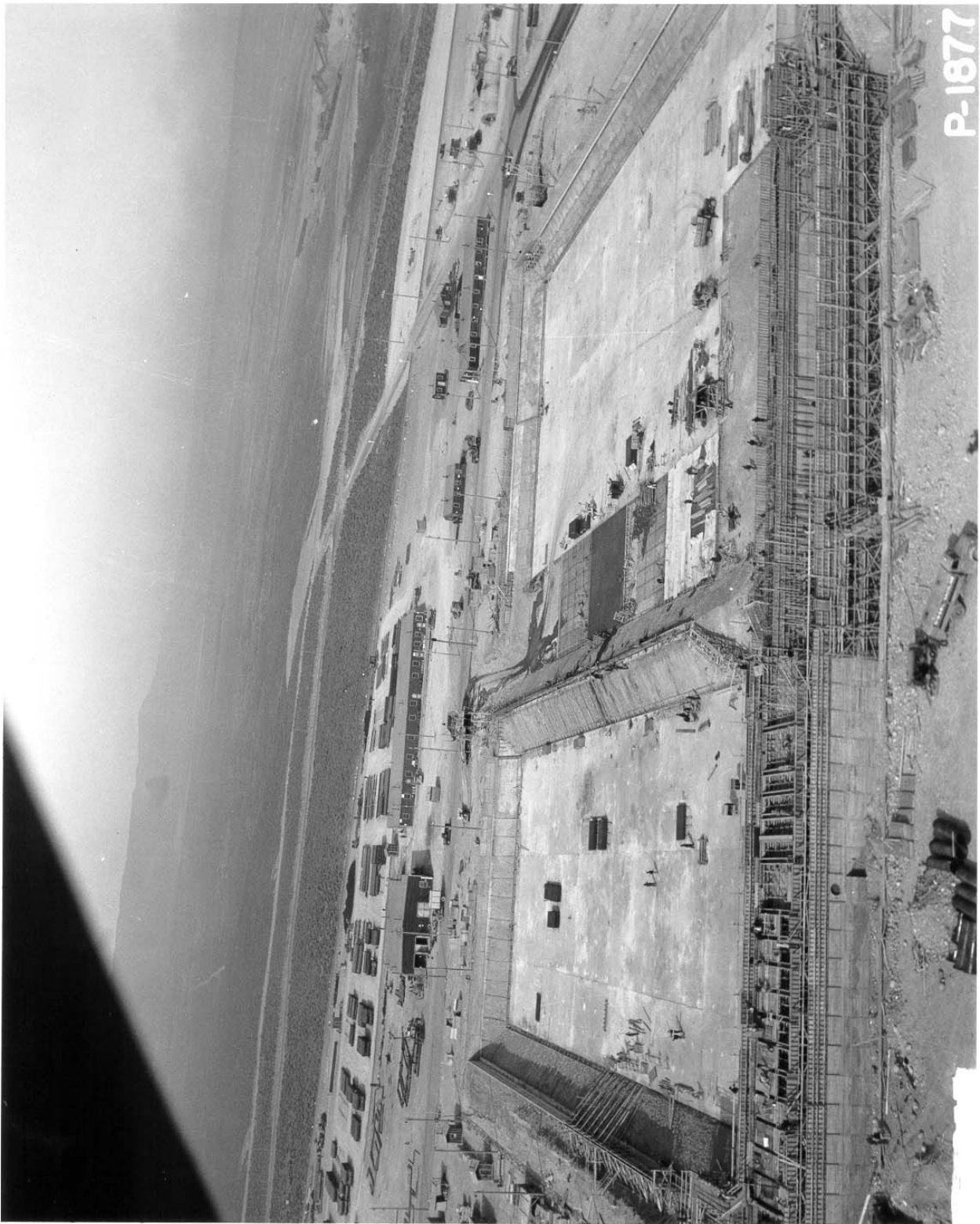
Photograph 14: The 182-B Reservoir under construction in March 1944, showing the divider which was normally covered by water. View is to the northwest. [P-1877]
