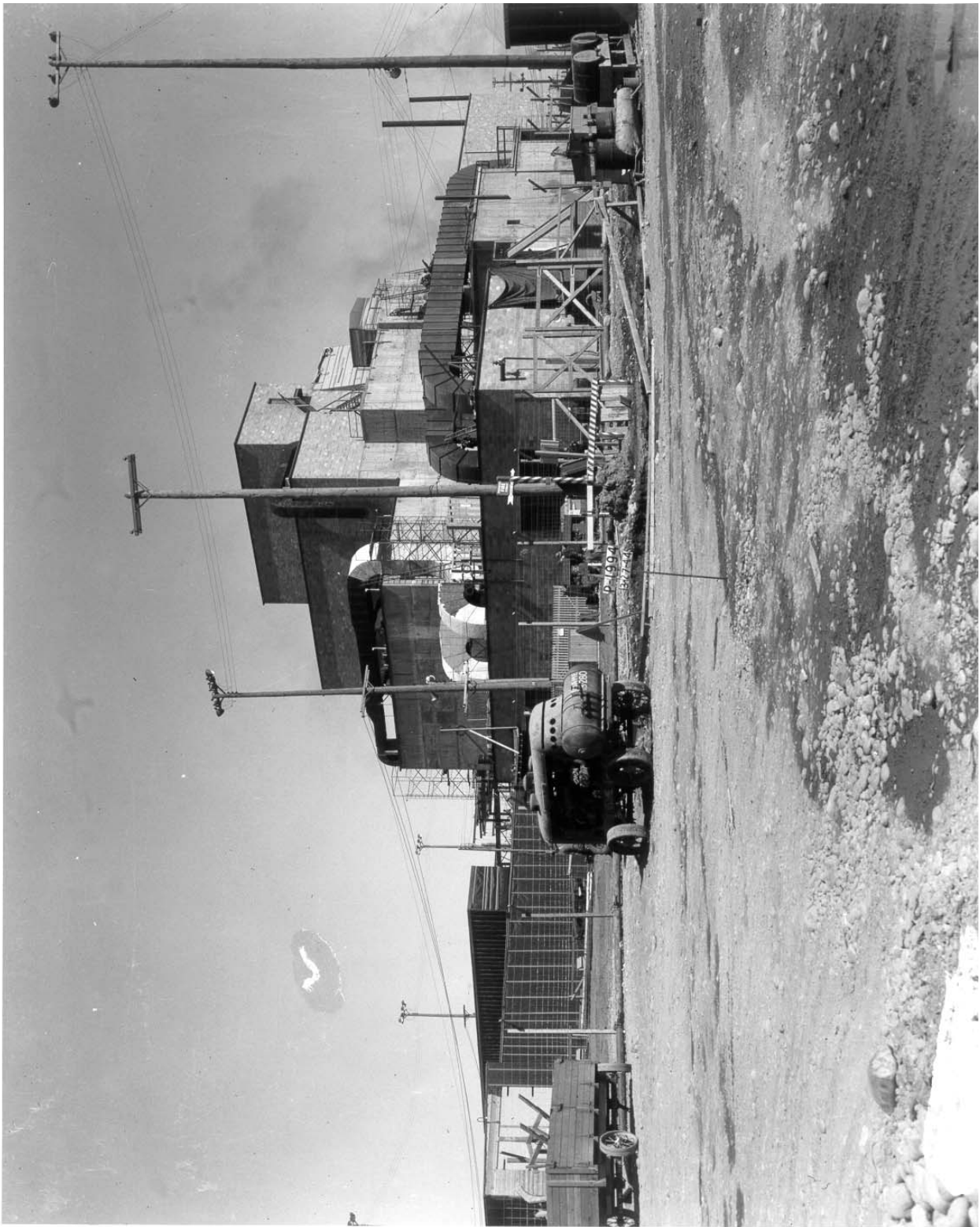
Photograph 3: The 105-B Reactor building under construction, with the exterior nearly completed except for the tall ventilation stack. [P-1994]
