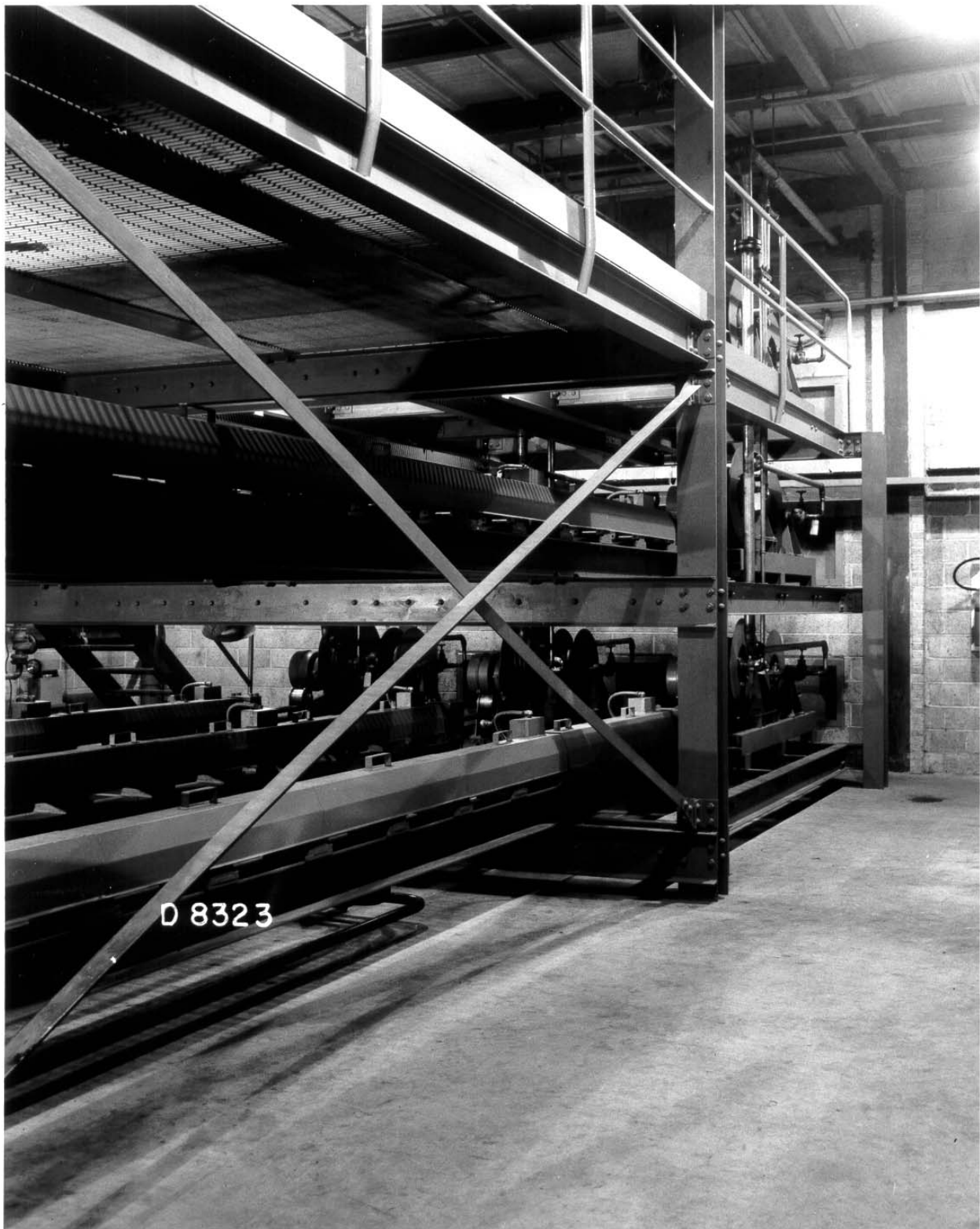
Photograph 26: A typical outer rod room, or rack room, showing the racks for the nine horizontal control rods (HCRs) that would be inserted or withdrawn from the pile to control the rate of reaction. In this case, it is in the 105-F Reactor in February 1945. The view is looking away from the pile, which is out of the picture on the left. Several of the cooling water hose reels for the rods can be seen at the end of the racks near the wall. [D-8323]
