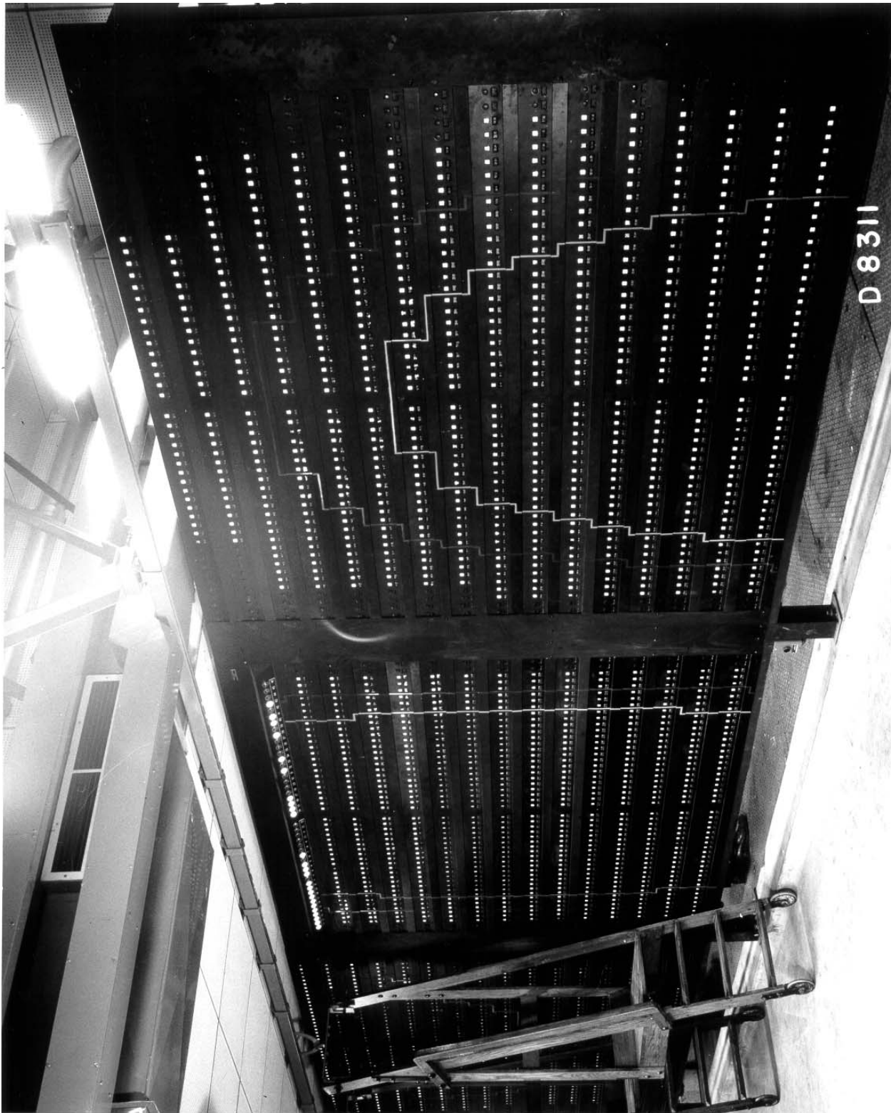
Photograph 29: An early picture of the Panellit gauges in the control room of a typical 105 reactor building, in this case 105-F in February 1945. There was one gauge for each of the pile's 2,004 process tubes. Each gauge monitored the tube's water pressure to ensure adequate cooling. Notice the wooden ladder, which operators could use when reading or adjusting the gauges. In later years, a large sign was installed across the top of the wall of gauges that read "Caution: Bumping This Panel Can Scram The Reactor." [D-8311]
