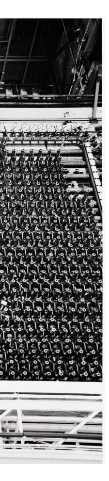
As you step through B Reactor's main entrance, pale-green double doors are visible straight ahead, at the end of a short hallway. It's behind those doors that B Reactor's atomic heart resides. In a vast, high-ceilinged hangarlike room, the enormous core looms 12 meters tall, its somber façade covered by protruding metal nozzles.
