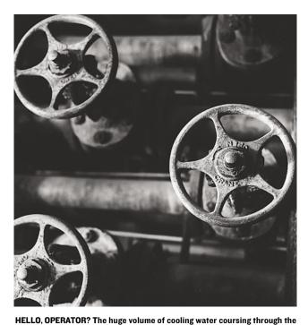
core created a deafening roar. Microphones [top] connected to loudspeakers were hung around the core to facilitate communication. Water flow through specific tubes could be controlled through a manual system of valves [bottom]. Uranium slugs removed from the core were put into special railroad cask cars that ran on tracks [opposite page] connecting the reactor to a chemicalseparation plant a few kilometers south, where plutonium-the reactor's end product—was extracted from the slugs.
