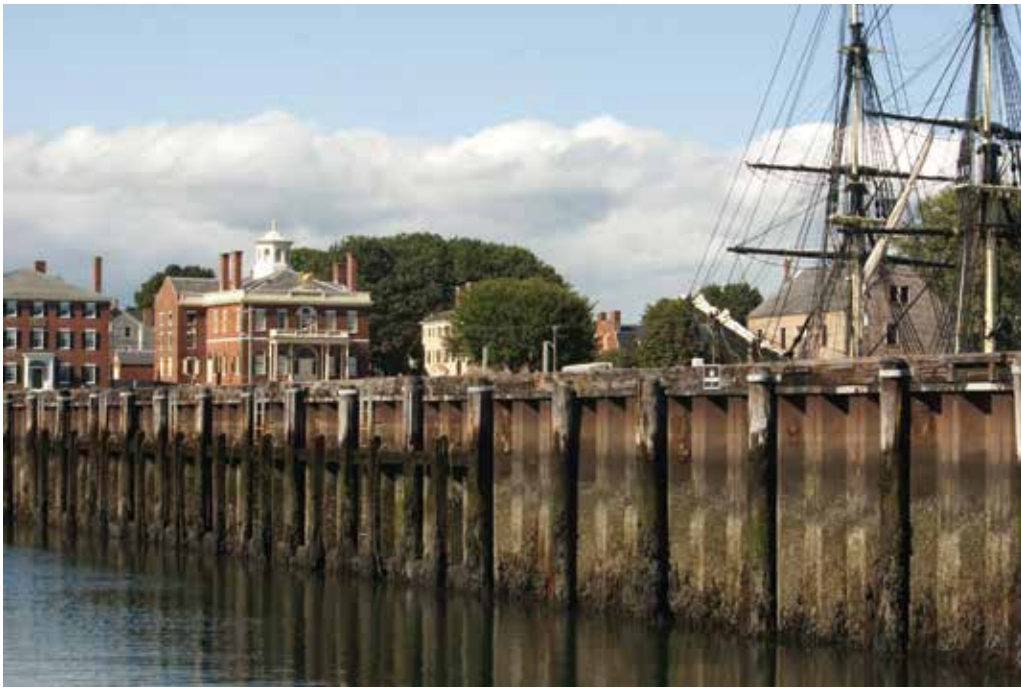
Salem Maritime National Historic Site, Salem, Massachusetts. Once more than 50 wharves extended into Salem Harbor. Three remain at the NPS historic site, which interprets colonial trade. Derby Wharf, built in 1806, is a half-mile long. The shorter Hatch's Wharf and Central Wharf were built in 1819 and 1791, respectively. The historic site includes some nine acres of land along the waterfront of Salem Harbor, including historic buildings, a replica of a tall ship, and the light station, built in 1871. Photo courtesy of the National Park Service.
