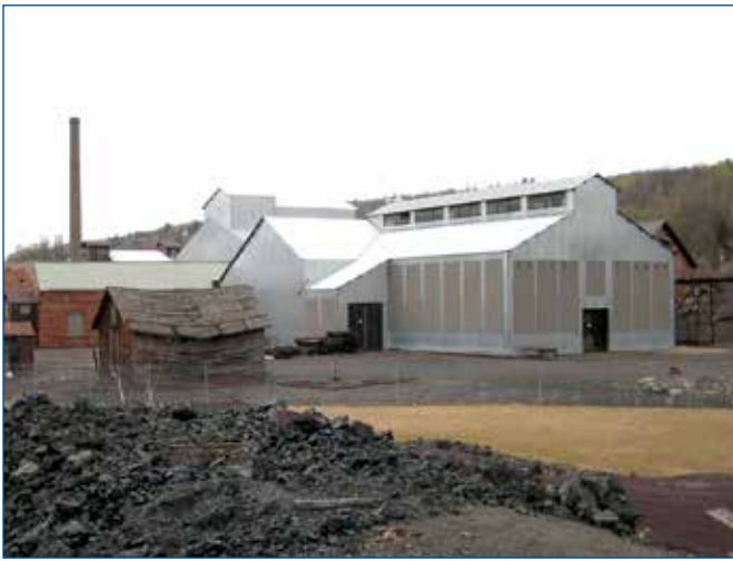
Figure 6: Casting Shed following stabilization, 2012. (source: Scott See)
