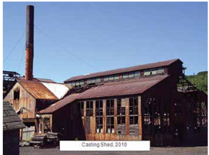
Figure 5: Casting Shed prior to stabilization, 2010. (source: Scott See).
