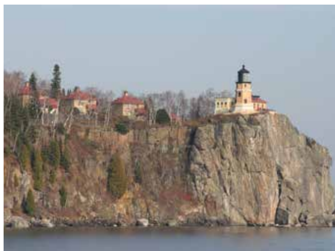
Split Rock Light Station, Town of Beaver Bay, Lake County, Minnesota. Built in 1909-1910 as part of a concerted effort to upgrade the Great Lakes navigation system, the Split Rock Light Station served the ports of Two Harbors and Duluth-Superior. From these ports, tons of iron ore were shipped to eastern industrial states and grain was shipped throughout the Great Lakes. The light station and associated buildings were designated a National Historic Landmark in 2011. Photo by John N. Vogel, October 2007; courtesy of the National Historic Landmarks Program.
