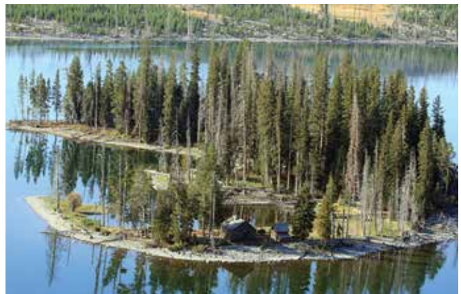
Historic Peale Island Cabin on Yellowstone Lake is threatened by shoreline change due to tectonic uplift. Photo from Coastal Adaptation Strategies: Case Studies , NPS.
