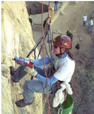
Applying silicon beading at Spruce Tree House.
