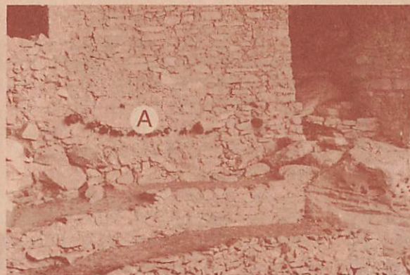
Original timbers; trash area
