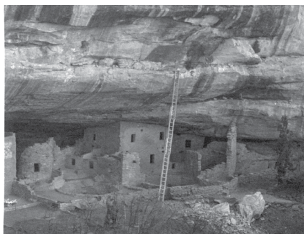
1960 rock fall. Note large debris field on lower right. One 10-ton rock fell, and a second, loose 5-ton slab was pulled down.
