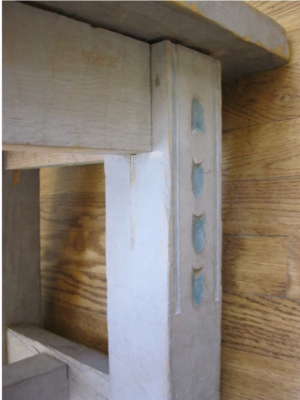
Photo 16 Close-up view of the color of a natural shale finish
