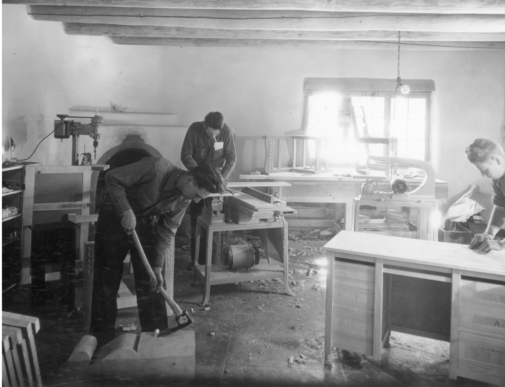
Photo 7 Historic photo, "Working in the improvised carpenter shop in the museum, Jan. 1936" (MEVE71372_171_989)
