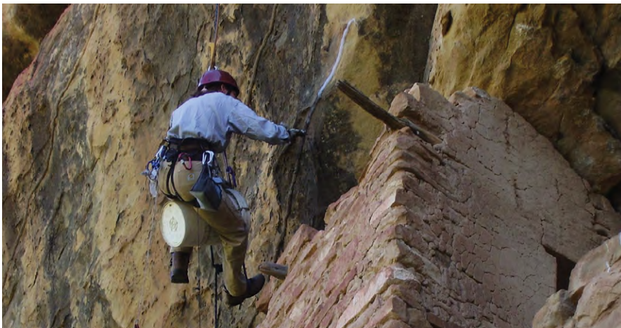
Cultural resource staff perform the preservation treatments needed to preserve the park's heritage resources in perpetuity. Here, a resource specialist rappels down a cliff face to lay silicon driplines. The driplines will direct runoff away from fragile architecture.
