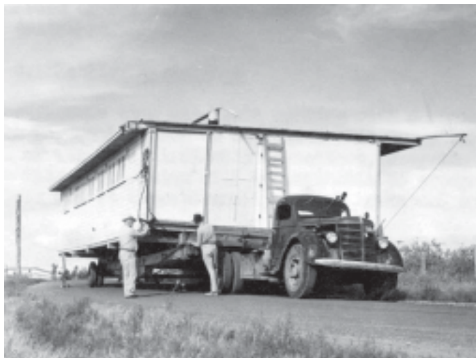
Moving a staff housing building to its new site in the warehouse area. Circa 1946. Photograph taken by Bureau of Reclamation staff. NPS Photo.
