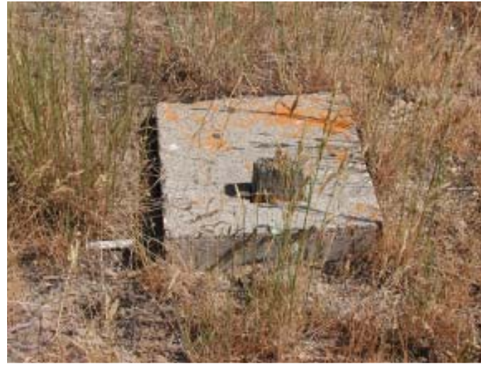
Building footing in the staff housing area. 2003. NPS Photo.
