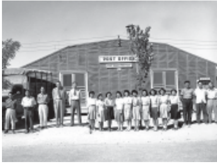
Minidoka post office in the administration area. Circa 1943. Permission of University of Washington.
