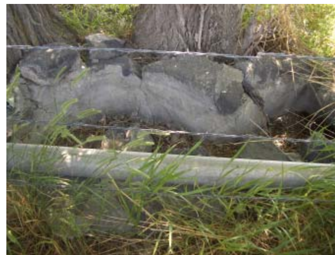
Historic fishpond, constructed by internees, along Hunt Road to the east of the national monument. 2003. NPS Photo.
