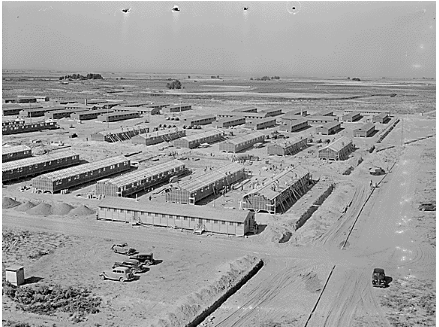
Minidoka Relocation Center under construction. Photograph by Francis Stewart. August 18, 1942. Permission of the Bancroft Library.
