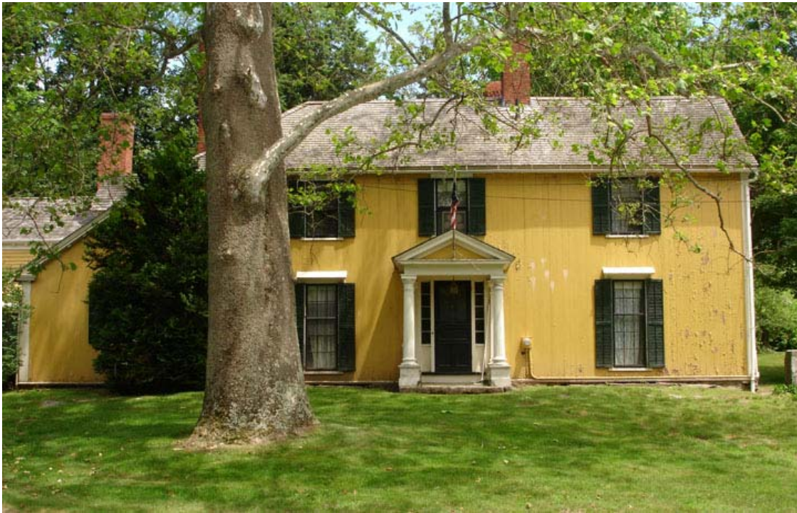
Figure 40. Elisha Jones House: West elevation (2006).
