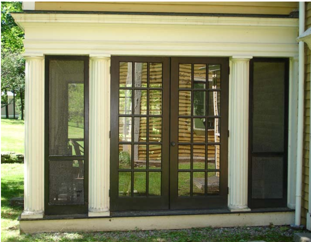
Figure 45. Elisha Jones House: North elevation of enclosed porch (2006).
