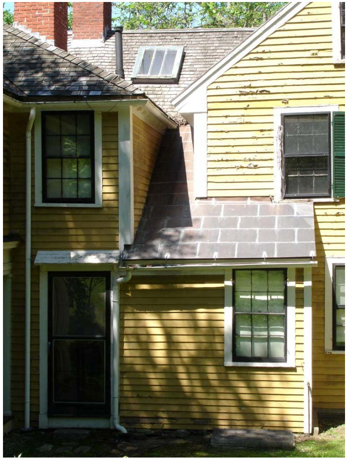
Figure 22. Elisha Jones House: East elevation, showing southeast hip roof (left) and north gable roof (right), with remnant of former lean- to roof kept as a valley between the two roofs (2006).
