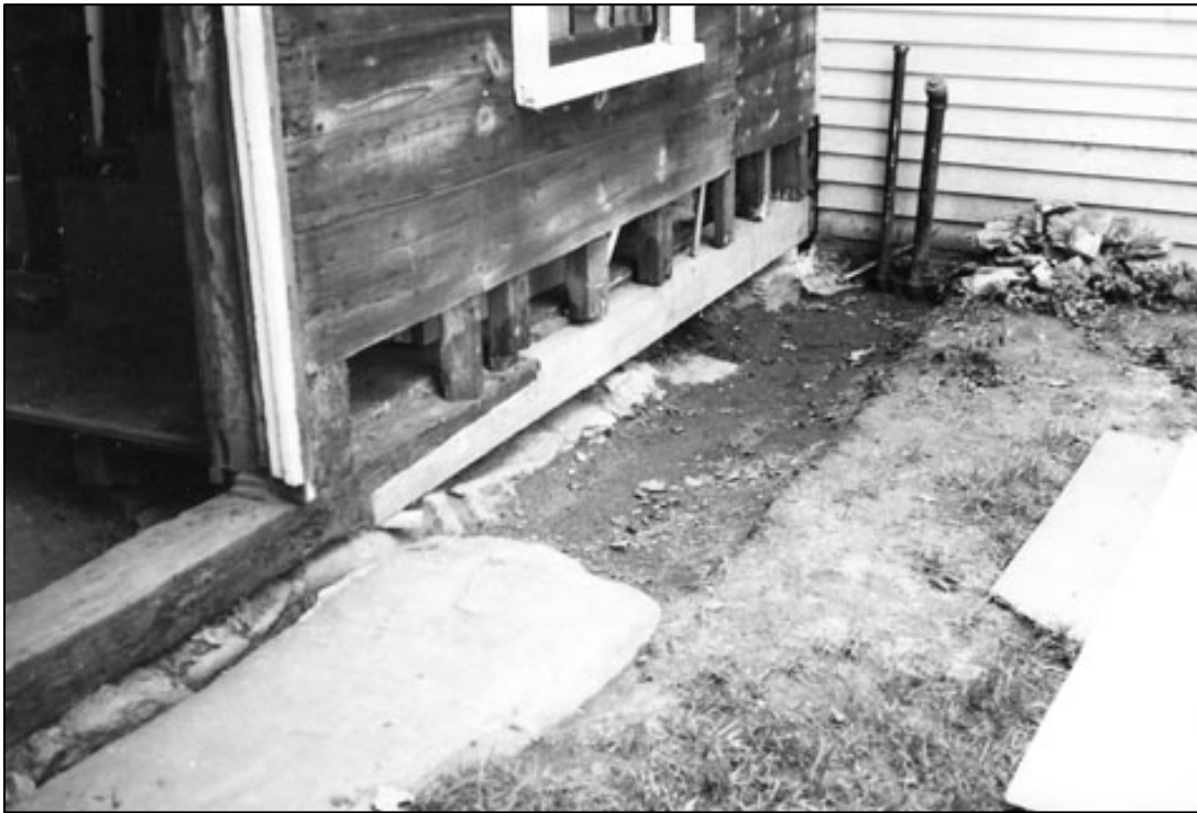
Figure 34. Elisha Jones Shed: West- wall sill repairs at south end of building, with a section of original sill (at left side of photograph) intact, 1974.
