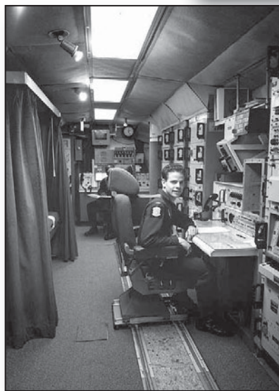
DELTA ONE LAUNCH CONTROL CENTER WITH CREW
