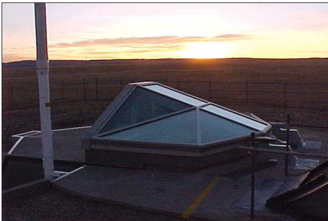
VIEWING ENCLOSURE OVER MISSILE SILO
