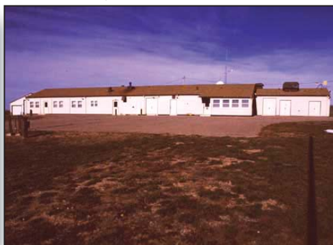
VIEW OF LAUNCH CONTROL FACILITY SUPPORT BUILDING, DELTA ONE
