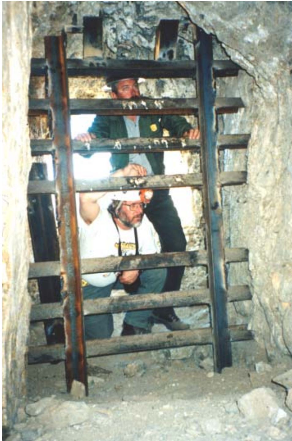
Figure 6. Inspecting bat gate at Sullivan Gold Mine, Joshua Tree National Park, California. (1999) Middle bar removed for access.
