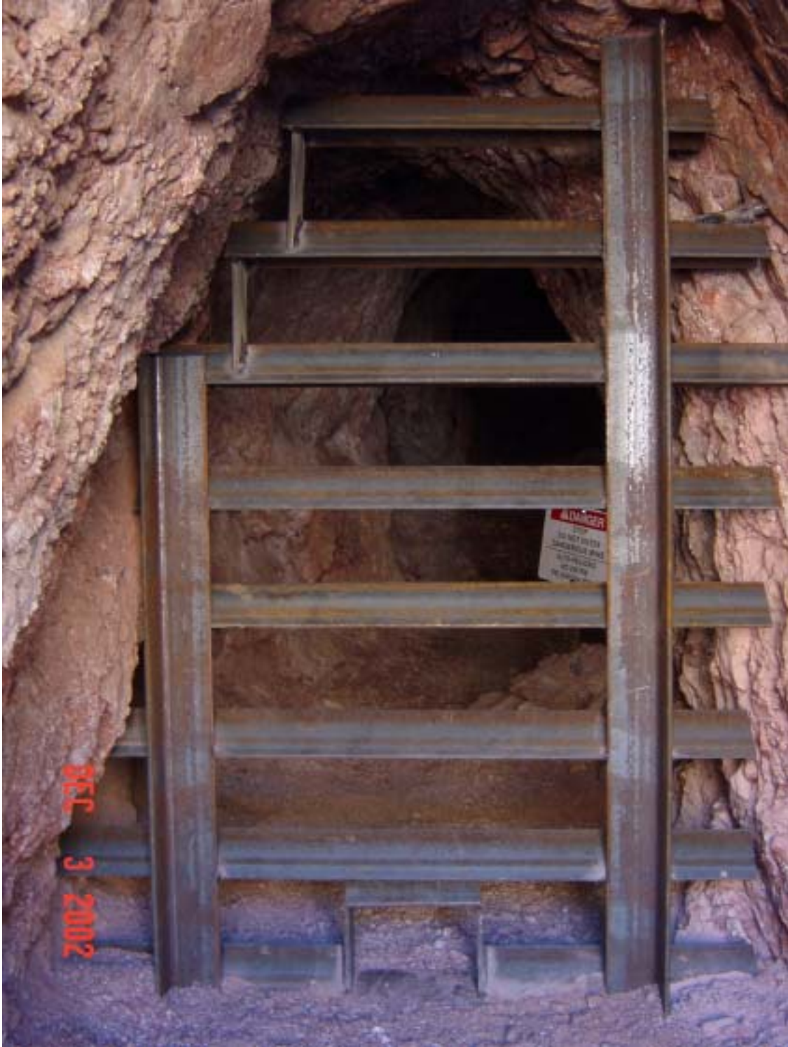
Figure 7. Bat gate at Katherine Access Gold Mine, Lake Mead National Recreation Area, Arizona. (2002) Note special access at base to accommodate desert tortoise, also known to use the mine.
