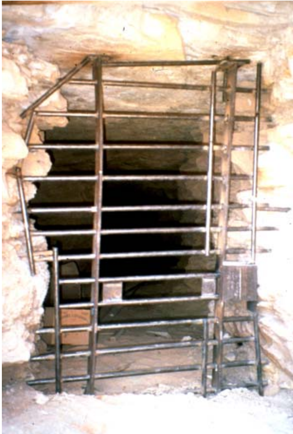
Figure 5. Manganal steel bar bat gate installed at Shafer Uranium Mine, Canyonlands National Park, Utah. (1998) Several perfectly-preserved wooden dynamite boxes dated 1953 were found in the mine, and were left within view of the gated entrance as part of the park's effort to interpret the mining history of the park.
