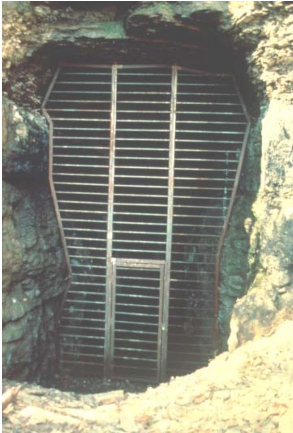
Figure 1. Bat gate installed at Kaymoor Coal Mine, New River Gorge, West Virginia. (1988)
