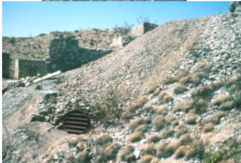
Completed bat gates at Mariscal Mercury Mine in Big Bend National Park. Note protective lock box for removable bar locking mechanism, and culvert gate used to maintain opening on unstable slope. This project was funded and contracted by the Railroad Commission of Texas Division of Surface Mining and Reclamation.
