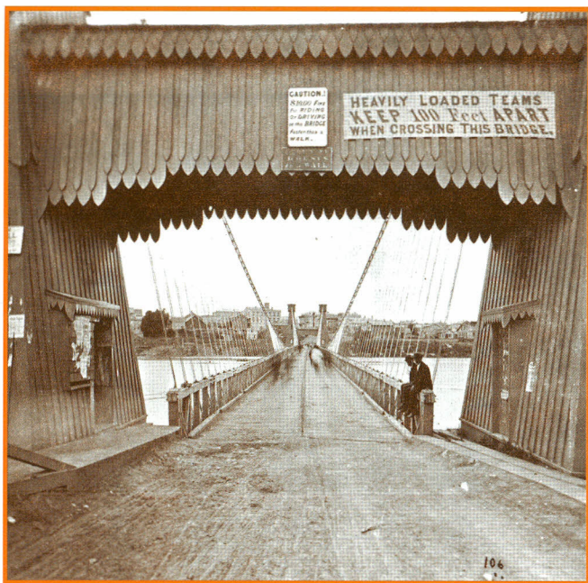
The first bridge ever to span the Mississippi River was completed in 1855, replacing the ferry. Built by private interests, it was a wooden suspension bridge with a roadway only 17 feet wide.
