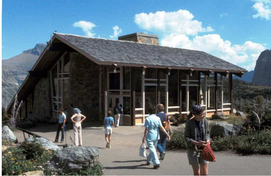
Figure 5.10. Western elevations of Logan Pass Visitor Center showing upper building with original window glazing, c.1977. The windows have since been replaced, with regularized placement of muntins and mullions. 193
