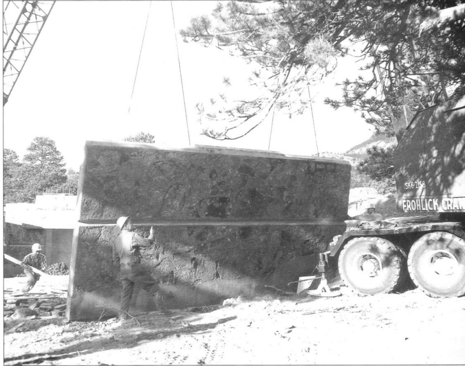
Figure 5.4. Precast stone and concrete panels being hoisted by crane, 1965. 166
