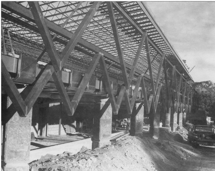
Figure 5.5. Exposed Cor-ten steel frame structure, 1966. 167
