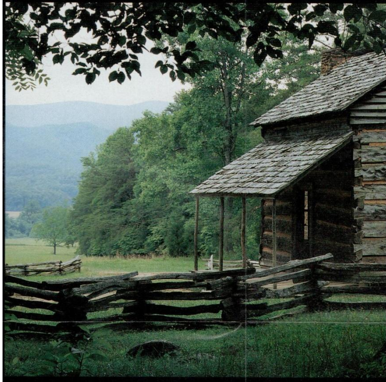
Figure 5.21. Example of log structures extant in GSMNP. 211
