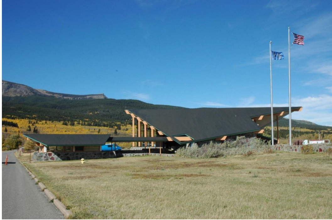
Figure 5.13. Southeast Elevation of St. Mary Visitor Center. 196
