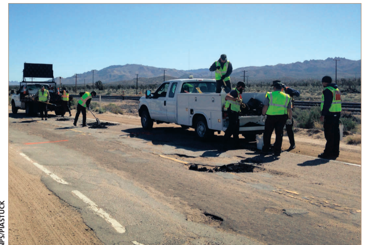
Mojave fire crew, rangers, office workers, managers, and other staff volunteer to fill potholes on Morning Star Mine Road.
