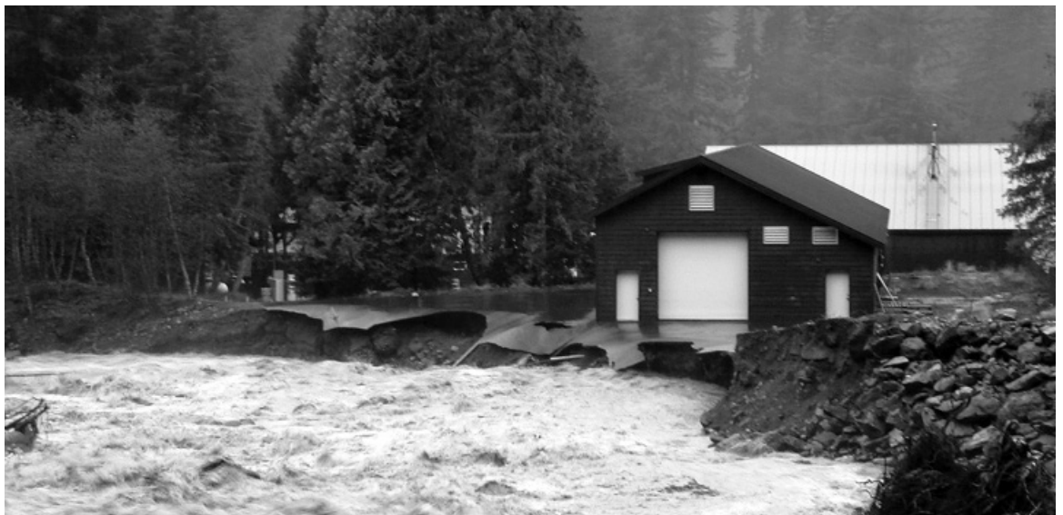
Damage to the Emergency Operations Center and protective levee at Longmire during the 2006 flood.
