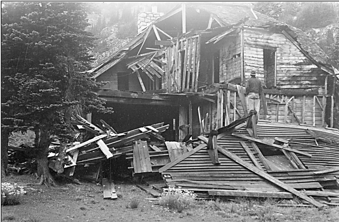
Figure 4.10. 1940-1942 Photograph of Glacier Basin Hotel after Partial Collapse in 1939. (MORA Archives)
