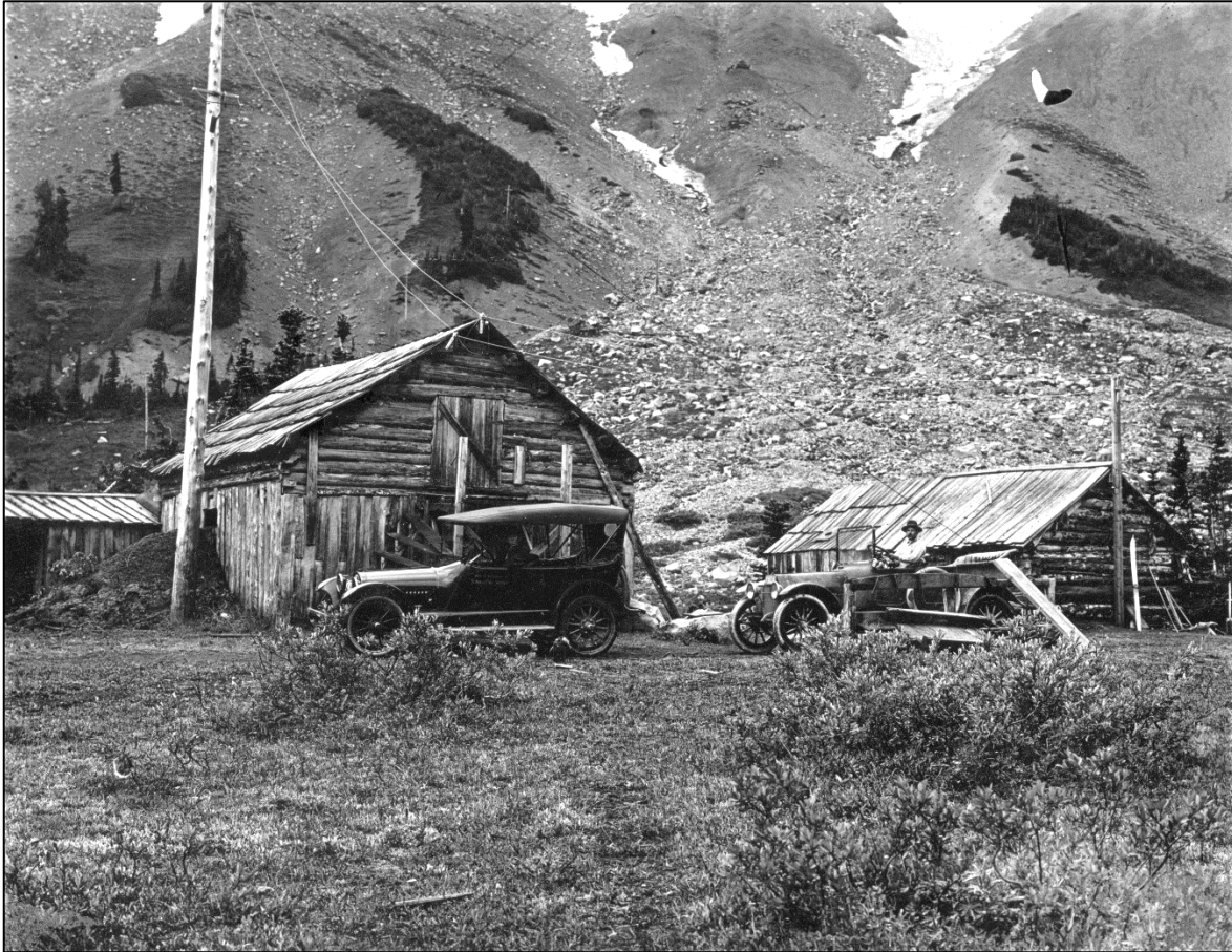
Figure 3.23. 1918 Photograph of Lower Camp's Barn ( left ) and Cabin ( right ). Barn with rear addition on the left with mound of manure and/or coal slag at side opening. Across the Inter Fork, the aerial ore tram is visible extending diagonally upslope behind the barn to Snowflake Lode. (MORA Archives)
