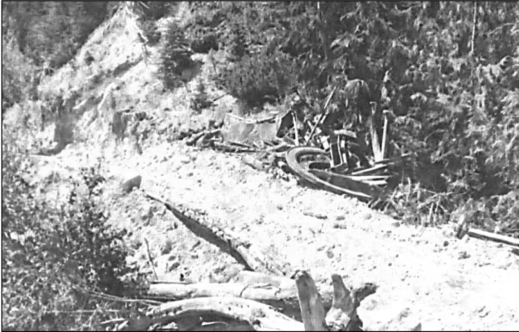
Figure 3.30. Ore Concentrator Parts beside Remains of the Storbo-Glacier Basin Road. (Photograph taken in 1952 by Douglas Evans. In NARA Archives L3023 Files Box 50 Folder 60)
