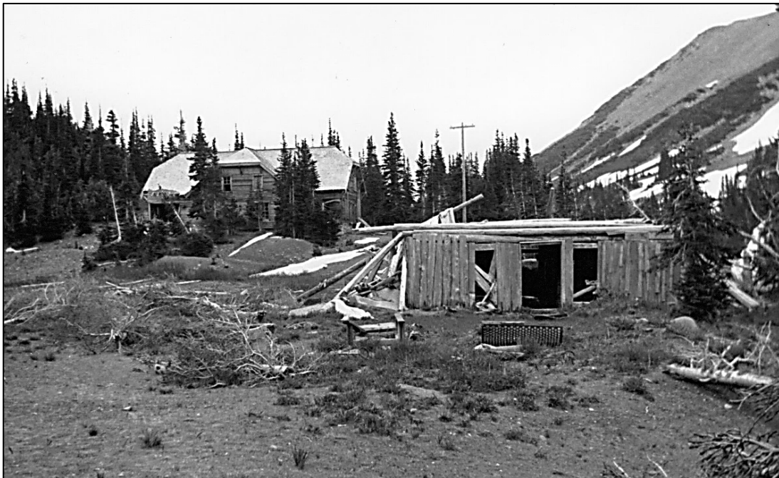
Figure 4.9. Deteriorating Lower Camp Structures in the 1930s. (Courtesy Arthur L. Storbo)
