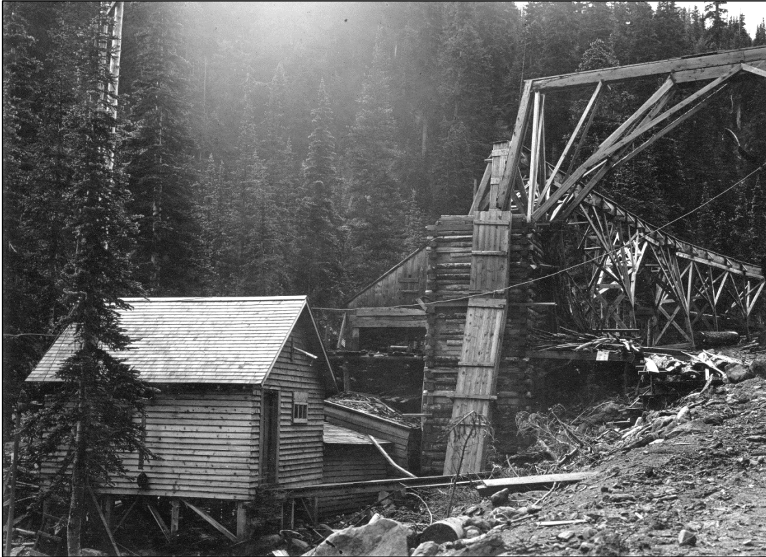
Figure 3.27. The Sawmill, Generator, Safety Breaker and Delivery Flumes Operating in 1918. (MORA Archives).
