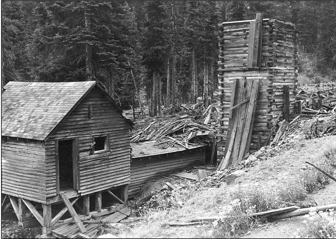
Figure 4.11. Glacier Basin Generator and Saw Mill ca. 1951.
