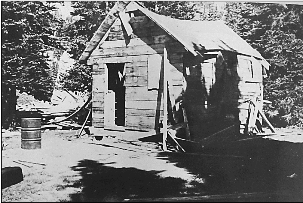
Figure 5.5. 12 by 14 ft. Shack Built in 1948 on the Storbo Hotel Site. Hotel ruins in background. 1951 Eastman report. (NARA Archives L3023 Files Box 51 Folder 59).
