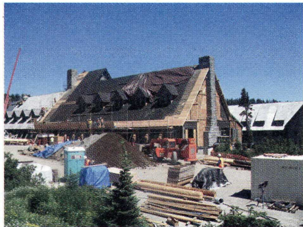
Rehabilitation of the historic Paradise Inn.
