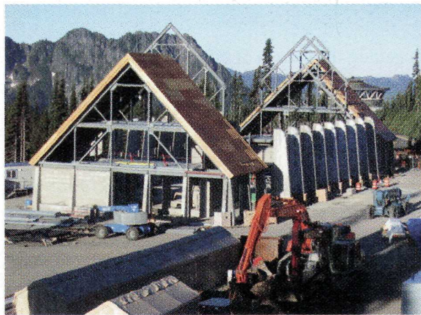
Construction of the new Paradise Visitor Center.
