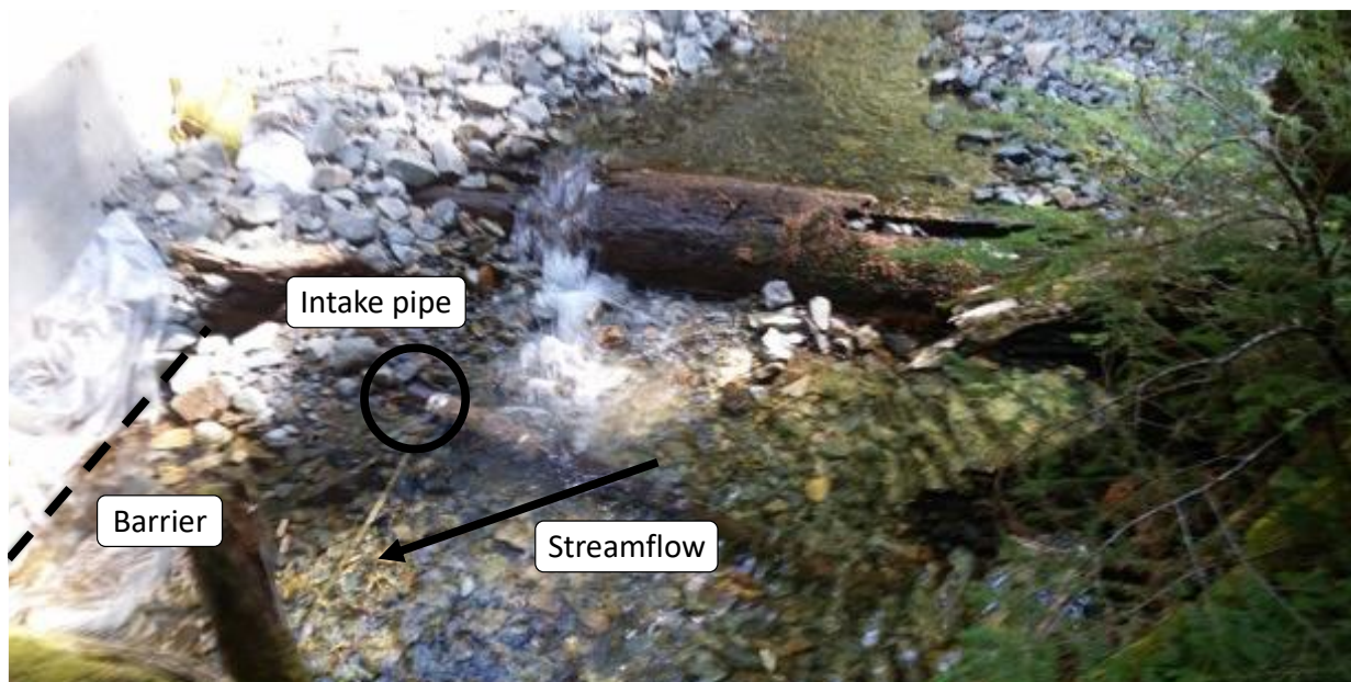
Figure 10. Photo of White River water intake positioned above water level on Klickitat Creek, August 28, 2015. Note the plastic barrier serving as the lower end of the impoundment on the left and arrow denoting the direction of streamflow.
