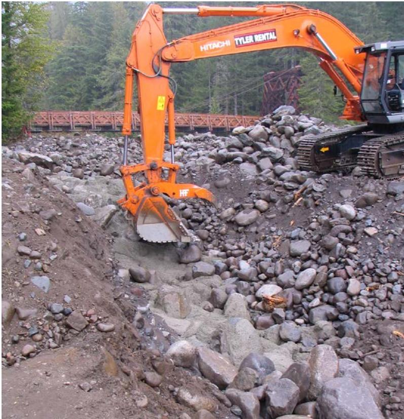
**Figure 26:** Construction of a flood wall in 2007 to help protect the Longmire administrative area from floods on the Nisqually River (Scott Beason/NPS Photo).
