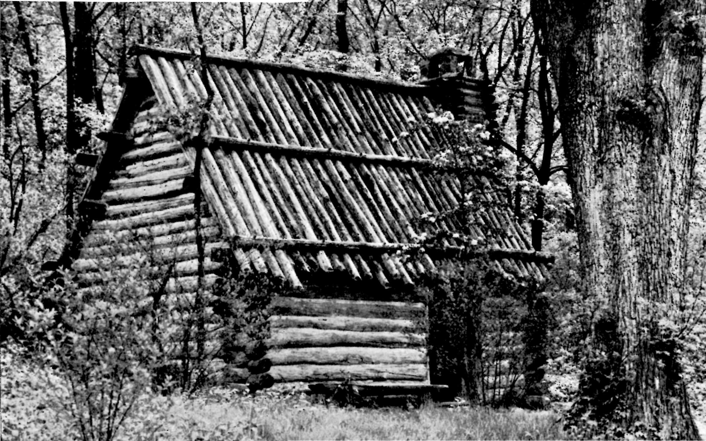
Reconstructed soldiers' hut in Jockey Hollow. About a thousand buildings of this type sheltered the Continental Army encamped near Morristown in 1779-80. The hut shown here is an approximate replica of an original structure which once stood on the same site. It is built of logs, chinked with clay, and fastened together with nails and wooden pegs. From 10 to 12 soldiers were billeted in each hut
