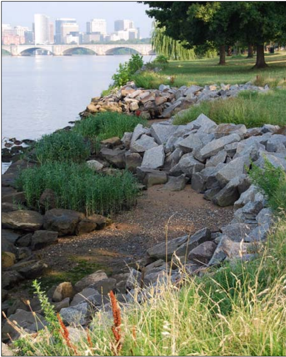
Riprap has been installed because of deteriorating rock walls.
