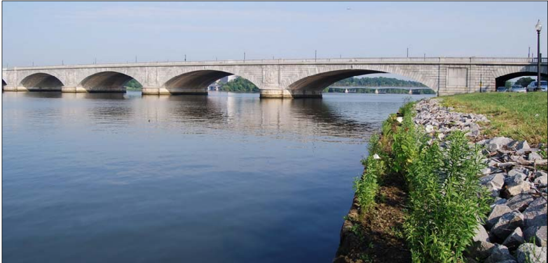
Riprap has been installed along sections of the Potomac River to stabilize the bank.
