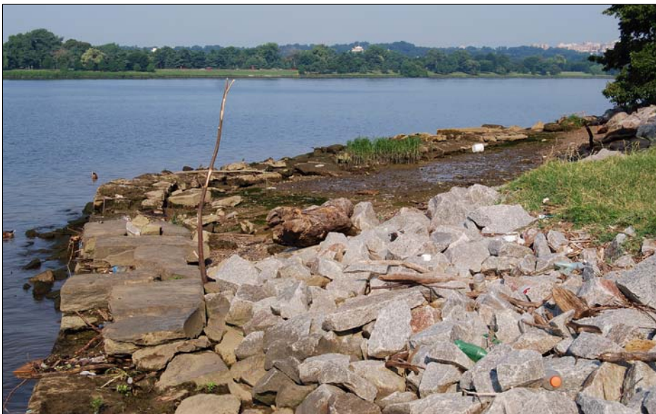
Looking northwest from near Inlet Bridge.
