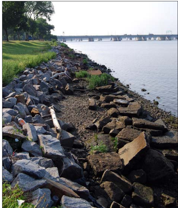
Riprap has been installed because of deteriorating rock walls.
