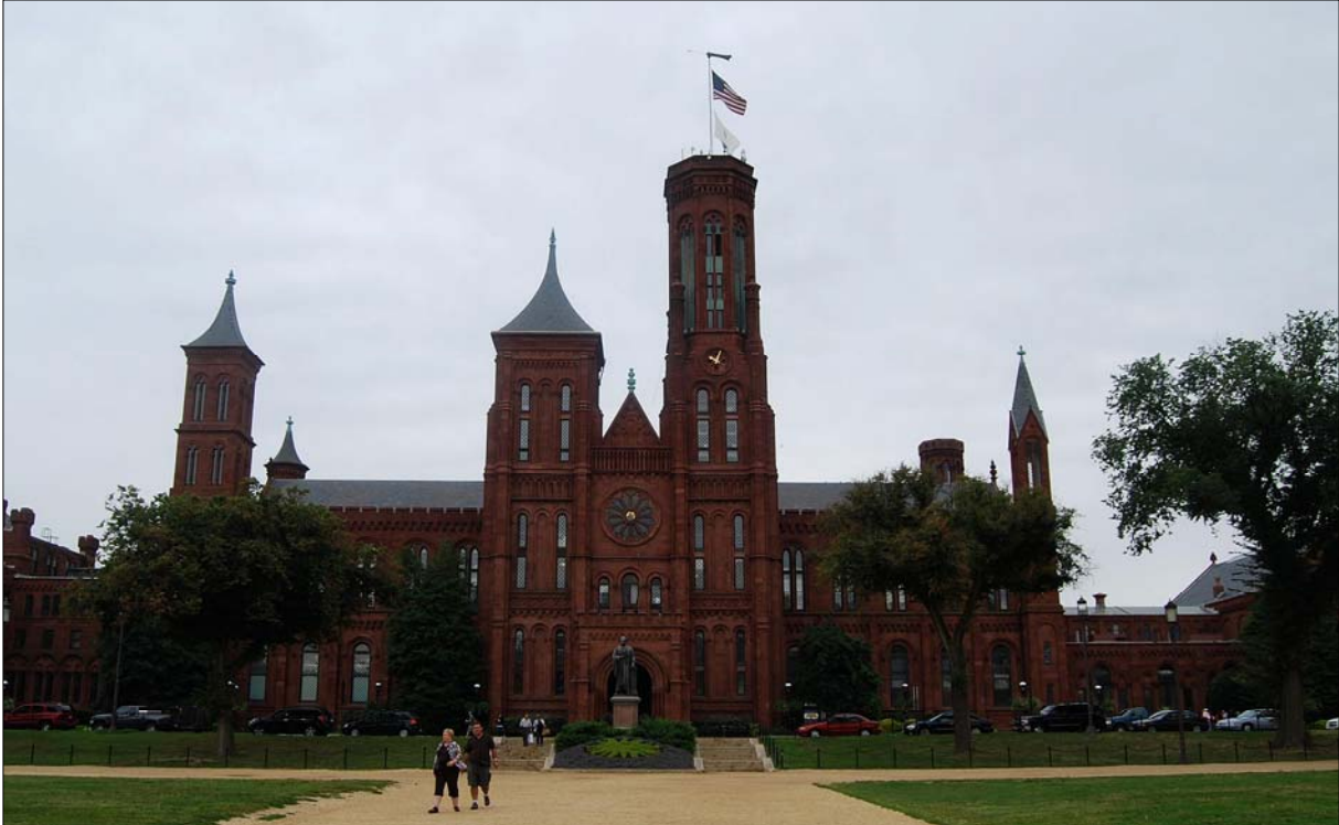
The Smithsonian Castle to the south. A security project for the Smithsonian Institution will move the Jefferson Drive closer to the center of the Mall.
