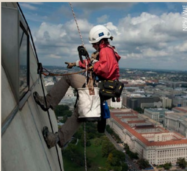
Structural engineer Emma Cardini inspects the Washington Monument's exterior, September 2011.
