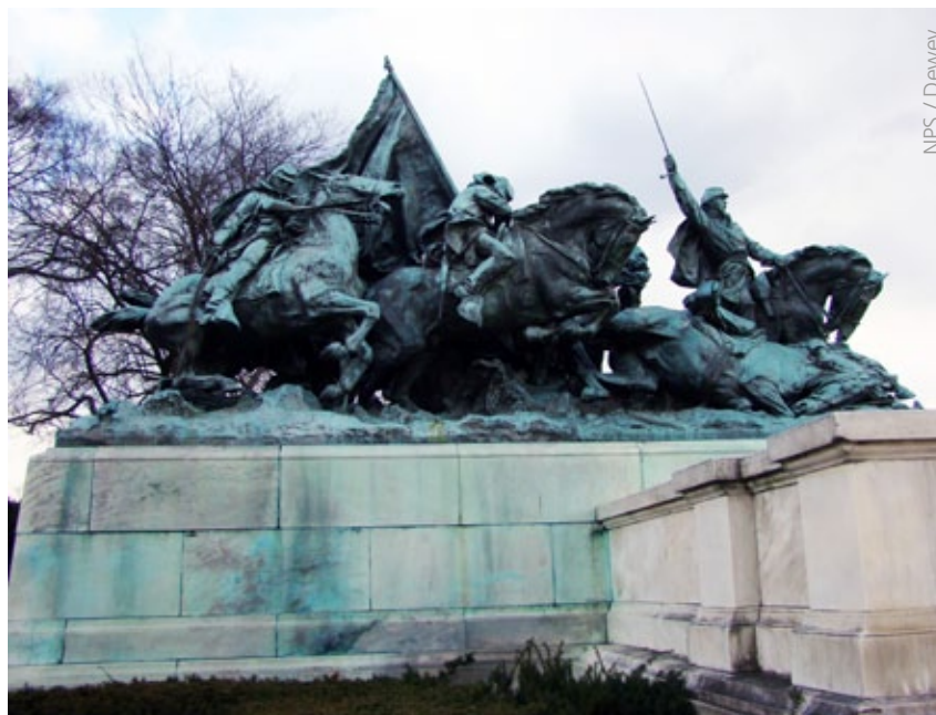
Green streaks on the base of the Ulysses S. Grant Memorial (on the west side of the Capitol Building) show where copper from the bronze statue, dissolved by acid rain, has stained the stone pedestal.
