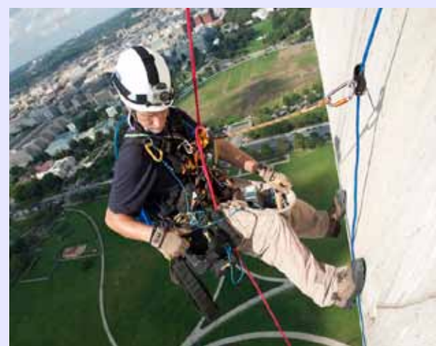
A structural engineer inspects the exterior of the monument.
