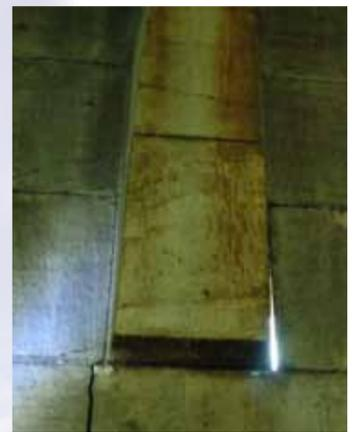
Daylight shines through a gap in the outer wall.
