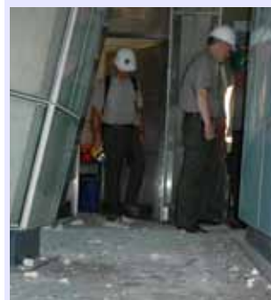
Debris fell within the observation deck as the building shook.
