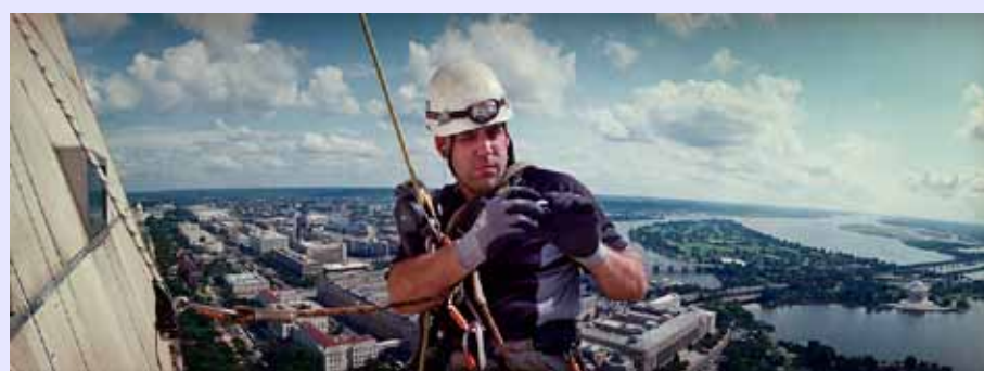
A structural engineer inspects the exterior of the monument.
