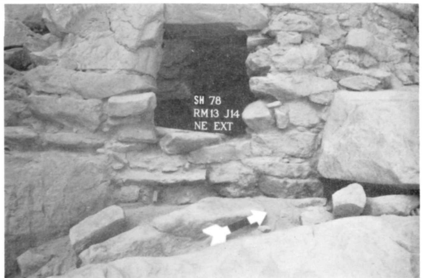
Figure 64. SHP-78 3-13-38. Room 13, job 14 northeast exterior wall after stabilization, June, 1978.
