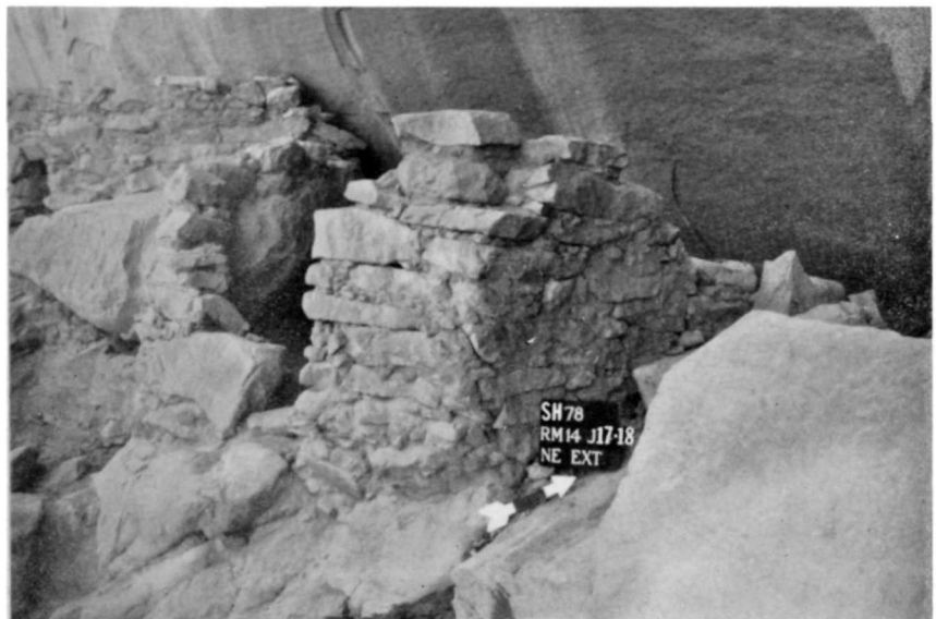
Figure 75. SHP-78 2-15-27. Room 14, job 17-18 northeast exterior wall after stabilization, June, 1978.
