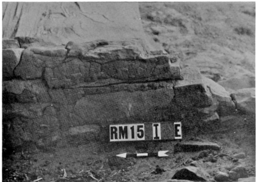
Figure 82. Room 15, job 21-22, before stabilization, August, 1977.
