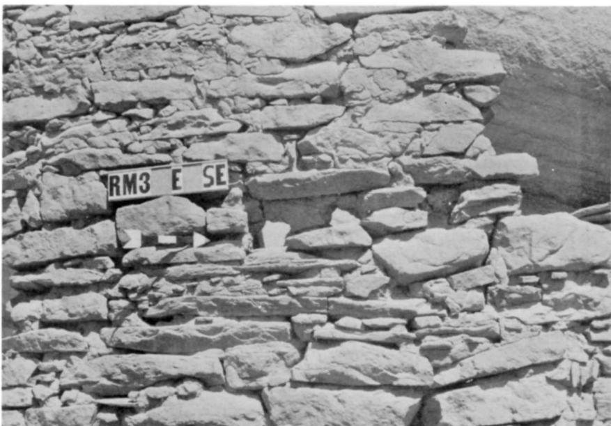
Figure 31. Room 3, job 2 before stabilization, August, 1977. Close-up.
