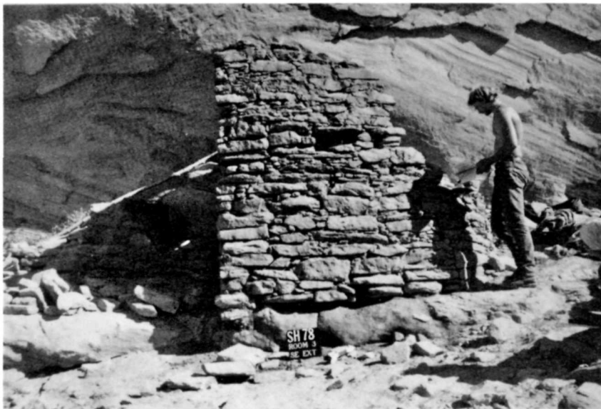
Figure 90. SHP-78 2-4-16. Room 3 southeast exterior after total stabiliza- tion, 1978.
