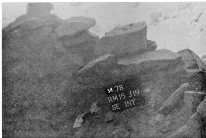
Figure 78. SHP-78 2-15-27. Room 15, job 19 interior of southeast wall after stabilization, June, 1978.
