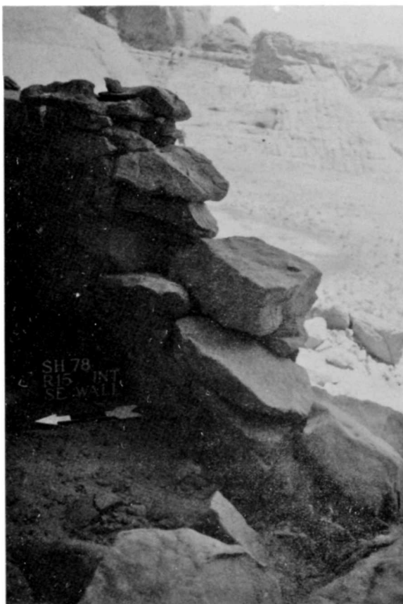
Figure 77. SHP-78 1-17-19. Room 15, job 19 interior of southeast wall before stabilization, May, 1978.
