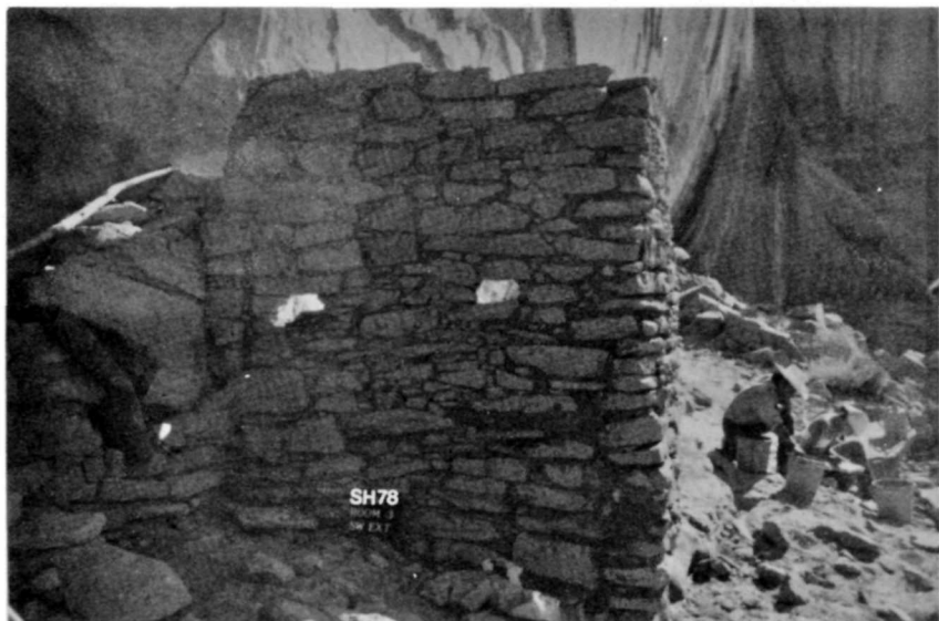
Figure 89. SHP-78 2-2-14. Room 3 south- west exterior after total stabilization, 1978.
