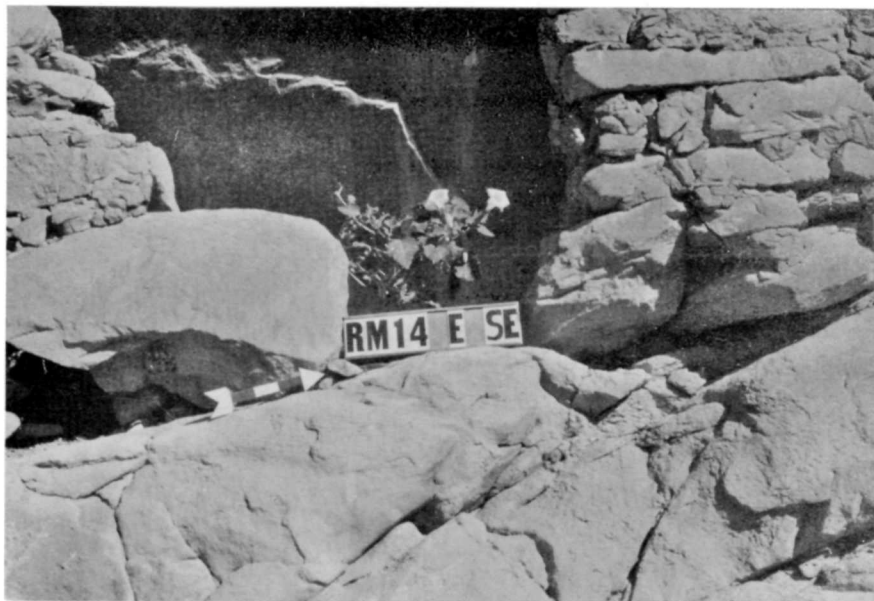
Figure 68. Room 14, job 16 before stabilization, August, 1977.
