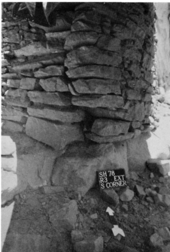
Figure 29. SHP-78 1-11-13. Room 3, job 1 south exterior of corner before stabilization, May, 1978
