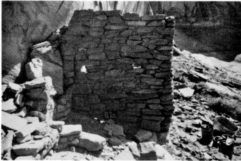
Figure 85. SHP-78 1-1-13. Room 3, job 23 southwest exterior wall before stabilization, May, 1978.
