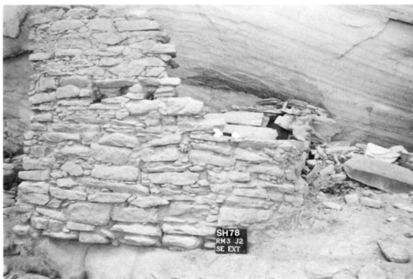
Figure 35. SHP-78 3-9-34. Room 3, job 2, south- east exterior wall after stabilization, June, 1978
