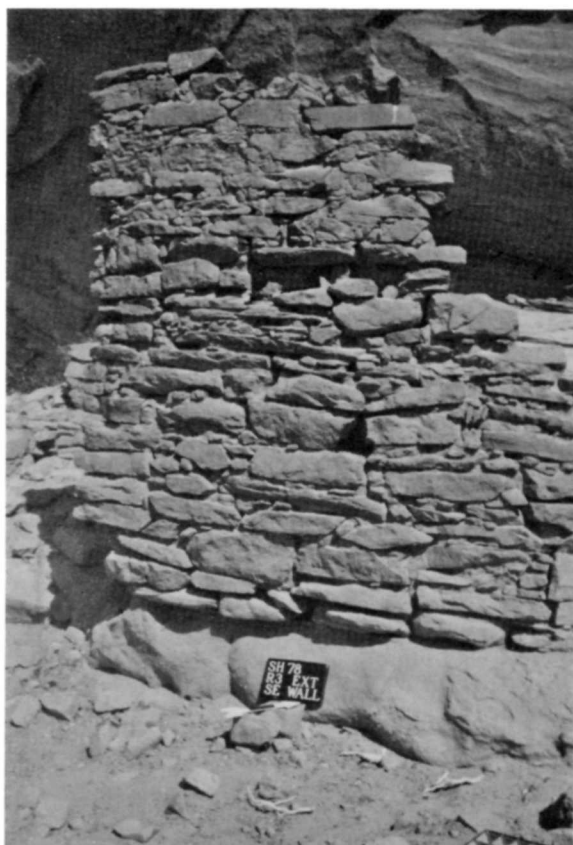
Figure 32. SHP-78 1-2-4. Room 3, job 2 exterior of southeast wall, before stabilization, May, 1978.
