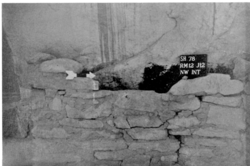
Figure 58. SHP-78 2-17-29. Room 12, job 12 northwest wall after stabilization, June, 1978.
