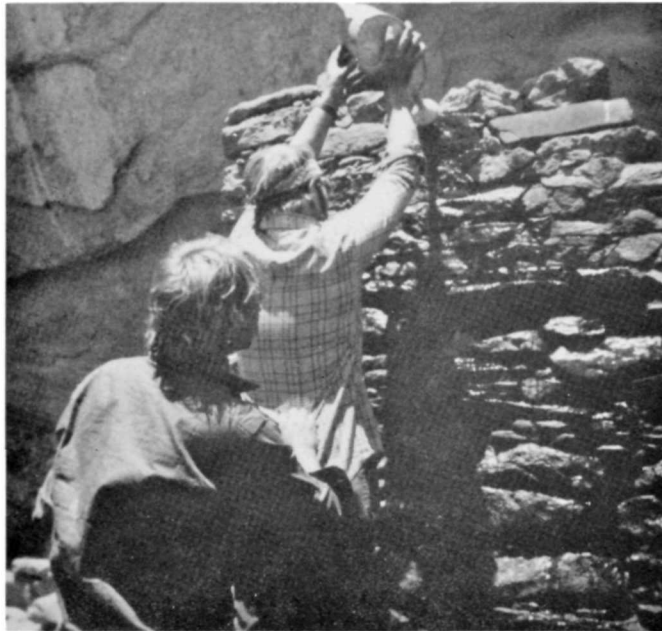
Figure 21. Second application of methyl methacrylate on highest portion of Room 3.
