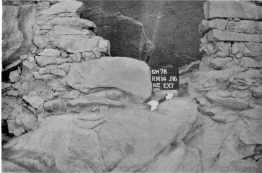
Figure 71. SHP-78 3-14-39. Room 14, job 16, exterior of northeast wall after stabilization, June, 1978.
