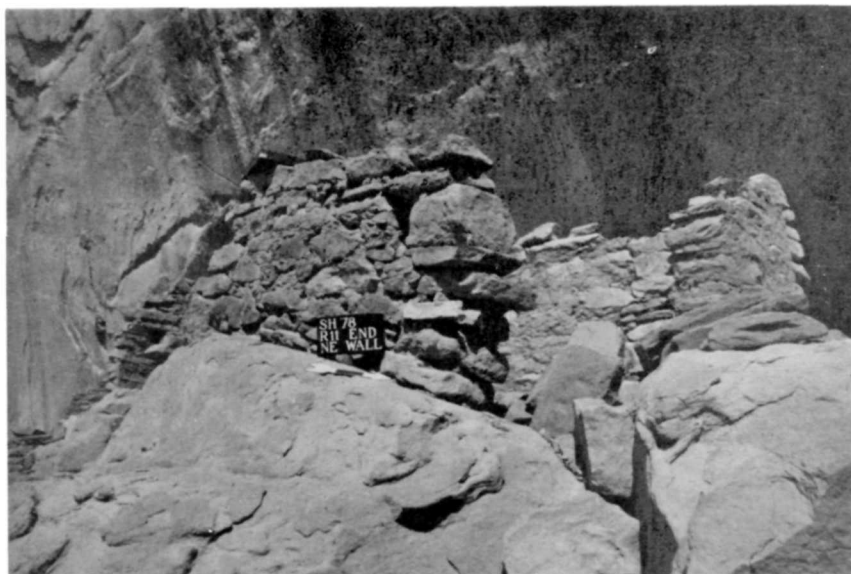
Figure 51. SHP-78 1-4-6. Room 11, job 9, northeast wall end before stabilization, May, 1978.
