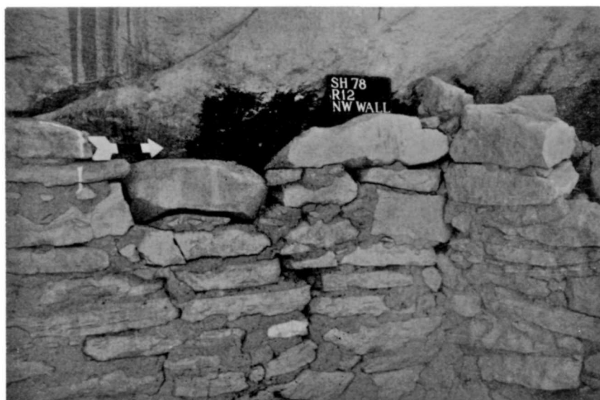
Figure 57. SHP-78 1-15-17. Room 12, job 12 northwest wall before stabilization, May, 1978.
