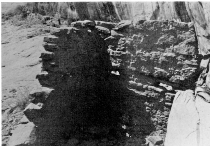
Figure 96. SHP-78 4-6-8. Winter check Room 3, southeast interior wall. Note position of sec- ond story floor beam seats. March 1979.
