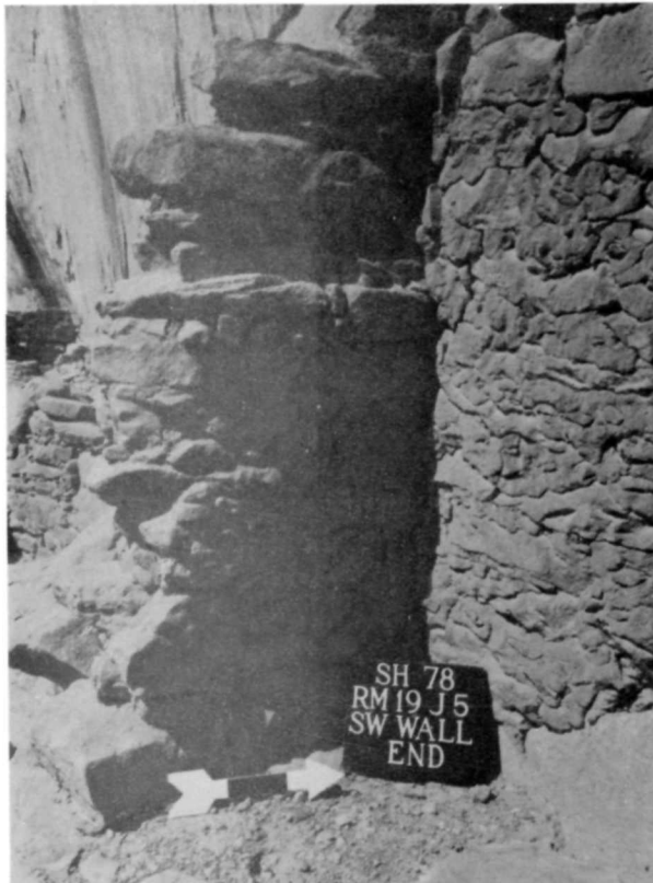
Figure 98. SHP-78 4-10-14. Winter Check Room 19, job 5; southwest wall end. Note water marking on mortar and stone. March 1979.
