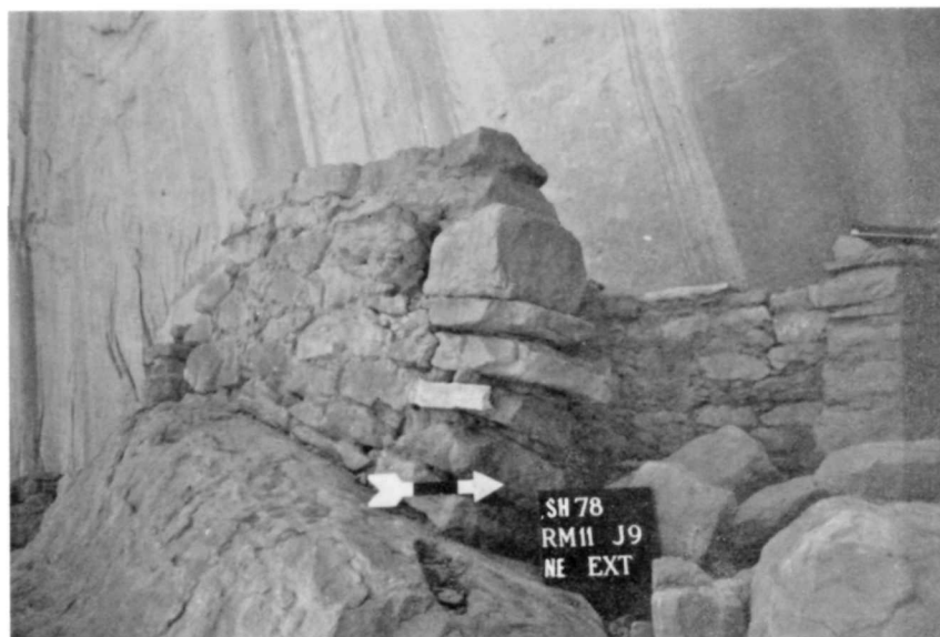
Figure 52. SHP-78 2-20-32. Room 11, job 9, northeast wall end after stabilization, June, 1978.
