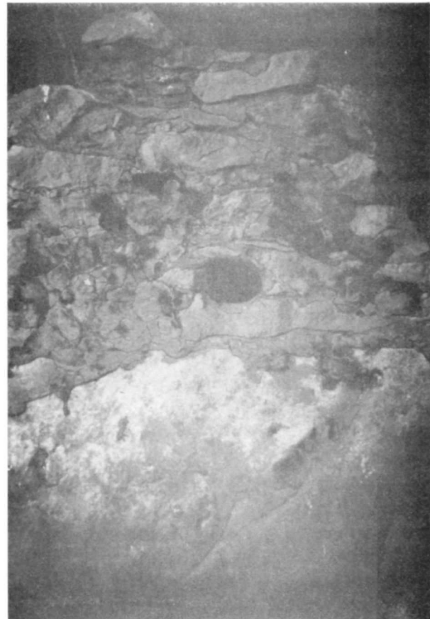
Figure 26. Example of plastering and niche in Room 15.
