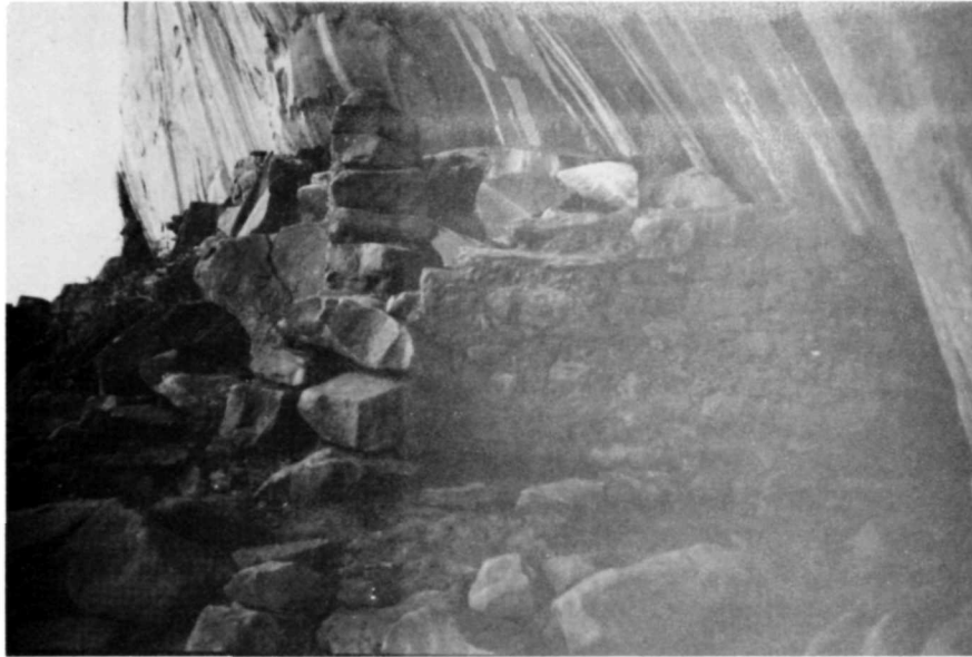
Figure 25. General view of the Kayenta masonry and techniques. Note uniform stone size, messy adobe and shallow nature of the overhang.
