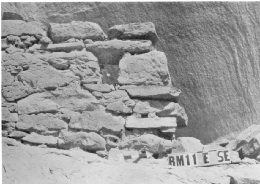
Figure 50. Room 11, job 9 before stabilization.
