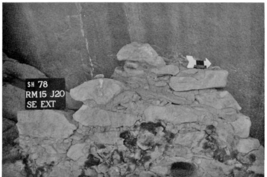
Figure 81. SHP-78 2-14-26. Room 15, job 20 exterior of southeast wall after stabilization, June, 1978.
