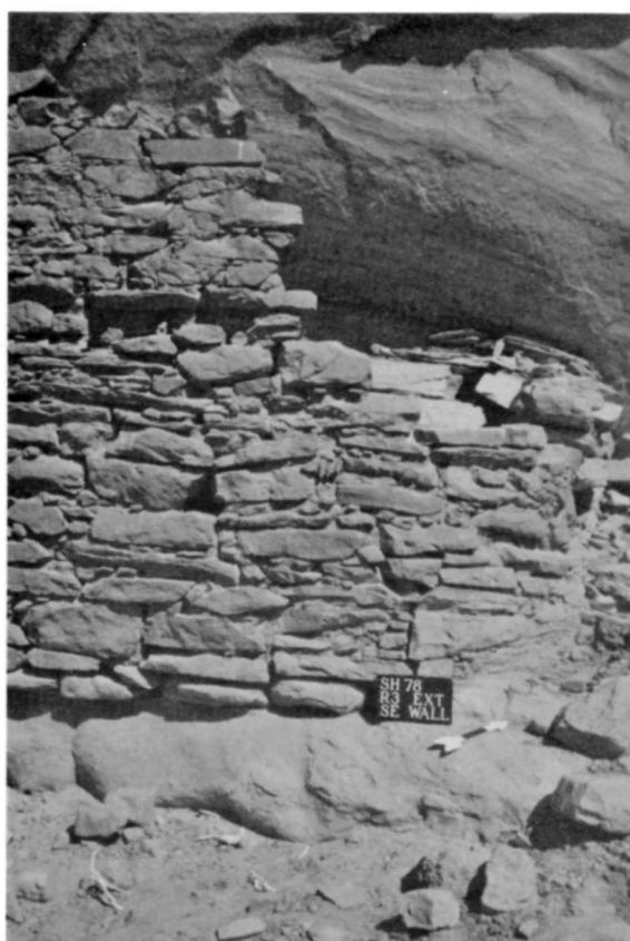
Figure 33. SHP-78 1-2-5. Room 3, job 2 exterior of southeast wall, before stabilization, May, 1978.
