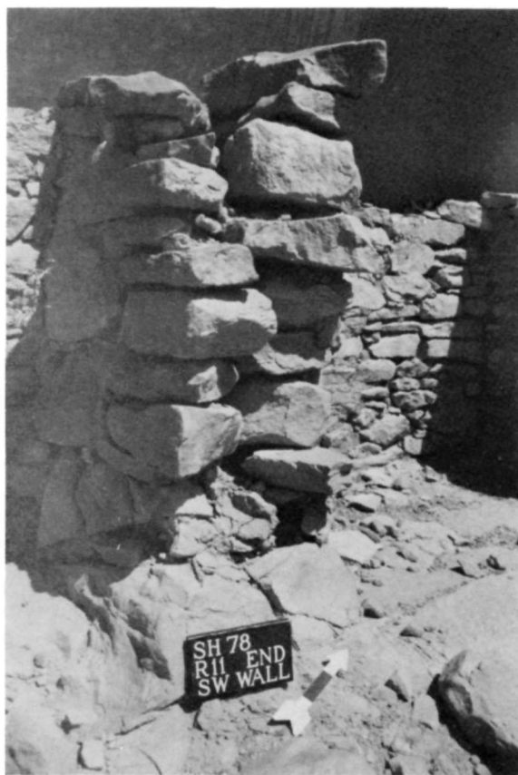
Figure 45. SHP-78 1-8-10. Room 11, job 6, wall end before stabilization, May, 1978.
