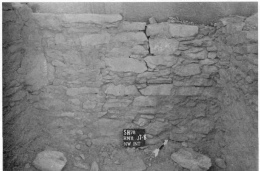
Figure 49. SHP-78 2-21-33. Room 11, job 7-8, interior of northwest wall after stabilization, June, 1978
