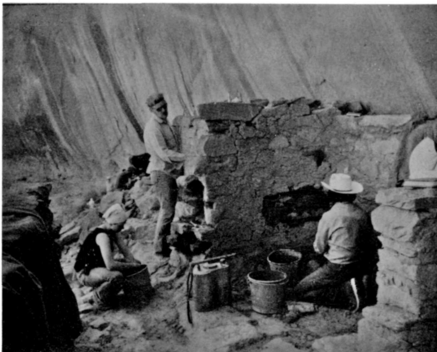
Figure 87. Room 11, job 24 during stabilization, May 1978.
