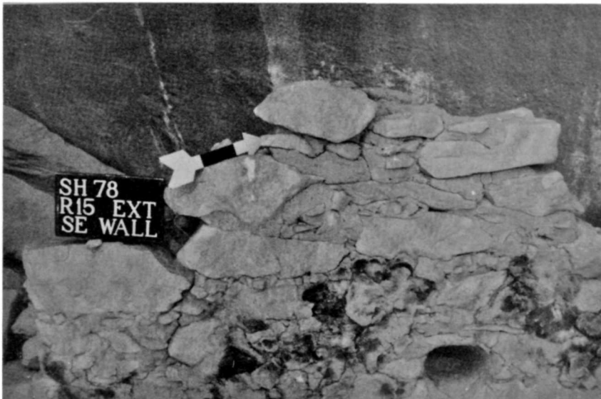
Figure 80. SHP-78 1-18-20. Room 15, job 20 exterior of southeast wall before stabilization, May, 1978.
