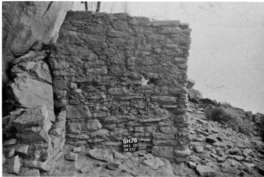
Figure 86. SHP-78 3-5-30. Room 3, job 23 southwest exterior wall after stabilization, June, 1978.
