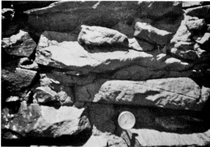
Figure 22. Close up of coated area still wet, and uncoated natural stone.
