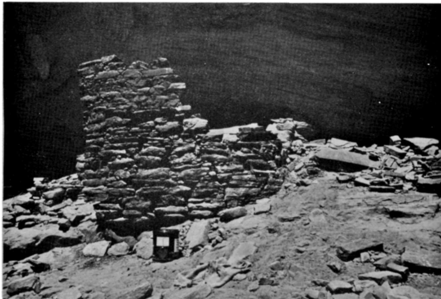
Figure 23. Room 3 after the final application of methyl methacrylate.
