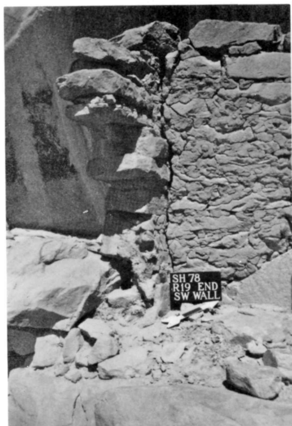
Figure 42. SHP-78 1-9-11. Room 19, job 5, southwest wall end before stabilization, May, 1978.
