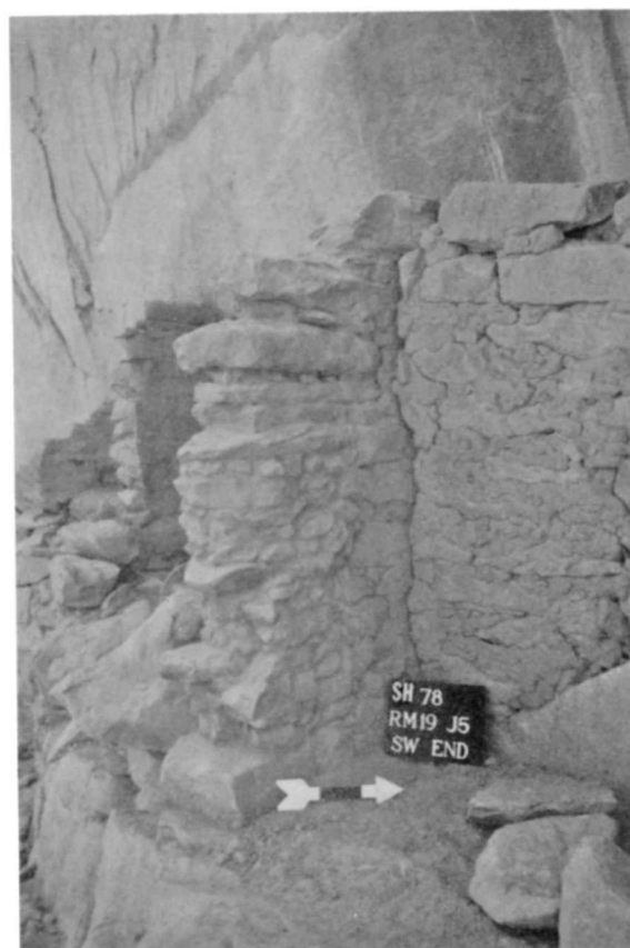
Figure 43. SHP-78 3-11-36. Room 19, job 5, southwest wall end after stabilization, June, 1978.
