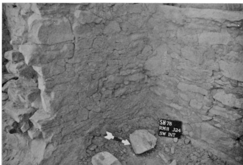
Figure 88. SHP-78 3-2-27. Room 11, job 24 southwest interior wall after stabilization, June, 1978.
