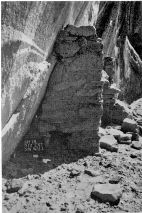
Figure 54. SHP-78 1-5-7. Room 12, job 10-11, southwest exterior wall before stabilization, May, 1978.
