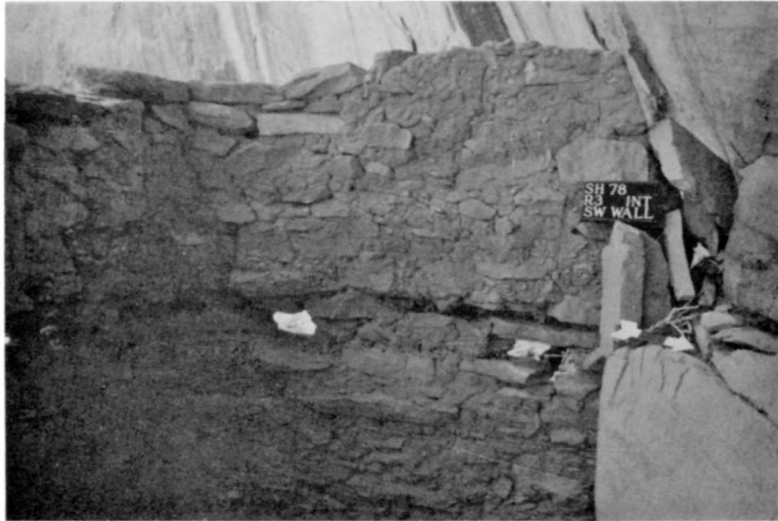
Figure 36. SHP-78 1-22-24. Room 3, job 3, Interior of southwest wall before stabilization, May, 1978.
