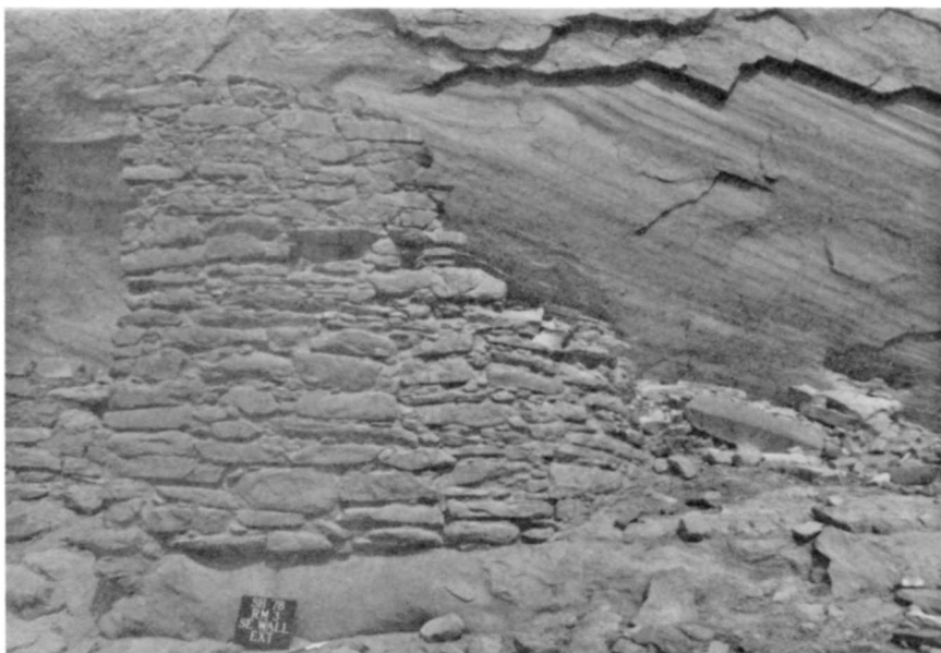
Figure 94. SHP-78 4-3-5. Winter check Room 3, southeast exterior corner. March, 1979.
