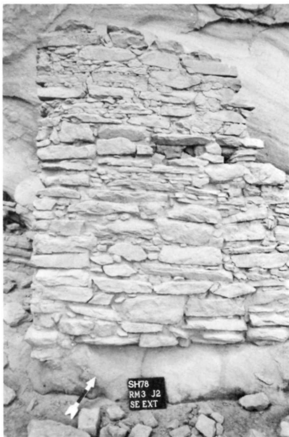
Figure 34. SHP-78 3-7-32. Room 3, job 2, southeast exterior wall after stabilization, June, 1978.
