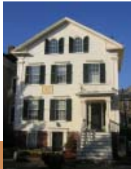
Nathan and Mary (Polly) Johnson House exterior rehabilitation is completed by the New Bedford Historical Society
