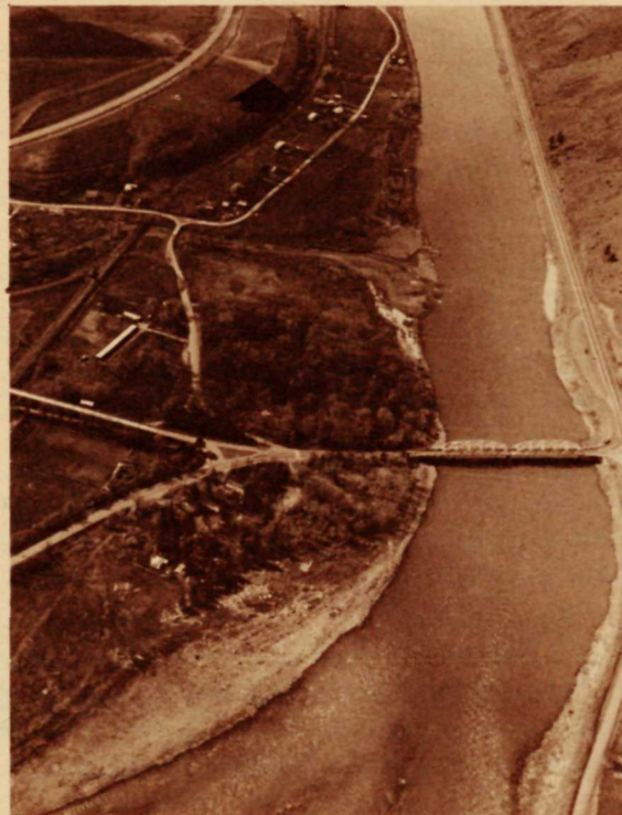
The Spalding area on the Clearwater River will accommodate the major interpretive facility and park headquarters. The Spalding Mission site of 1838-47 is located in the treed area, center. The interpretive and headquarters area will be located on the ridge adjacent to the worn area, arrow.
