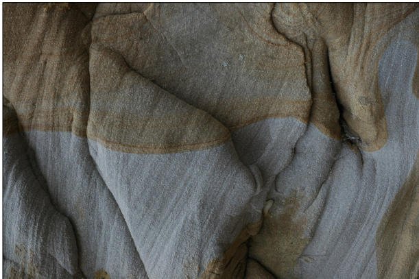
Railroad workers often had to cut through walls of sandstone to complete line construction, like this stone on the Rend Line, which was finished in 1904 near Thurmond. Photo by Jodi French-Burr.
