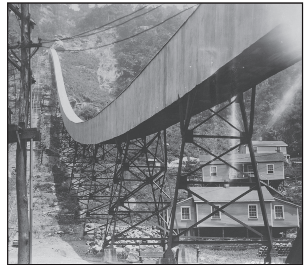
Henry Ford installed a $100,000 conveyor system called "button and rope" that was designed for gentler transport of coal. From the collections of The Henry Ford.
