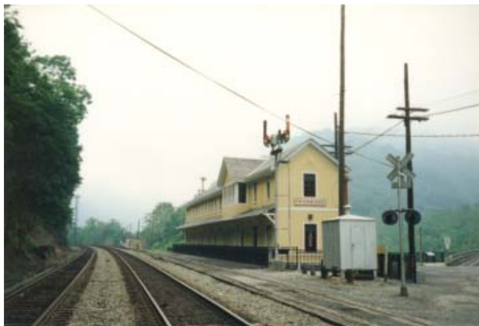
The restored train depot (located in the Thurmond Historic District).
