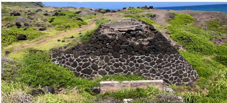
Stonework of a remaining railroad trestle at Ka'ena Point State Park, Mokulē'ia section | Nā pāpōhaku i koe mai nā hūlili alahao i koe ma ka Pāka Moku'āina o ka Lae 'o Ka'ena, ka māhele 'āina o Mokulē'ia
