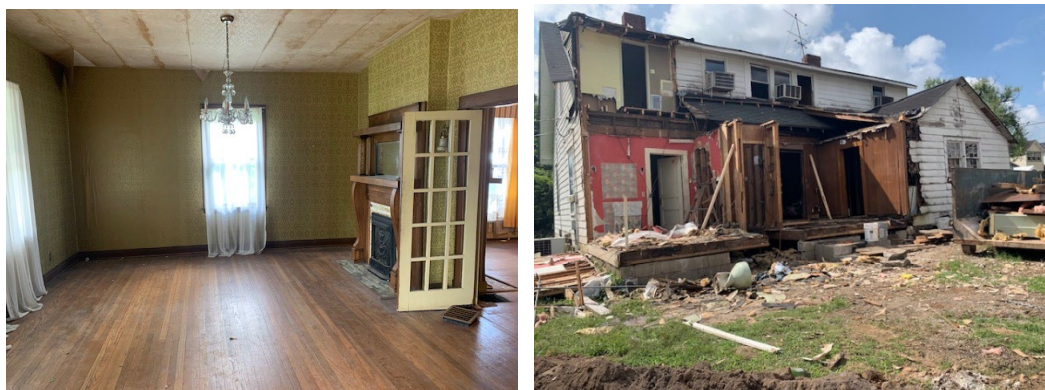
Restoration underway at Merrill-Williams House, Franklin
