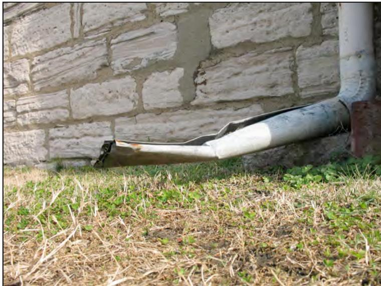
Some of the lower gutter sections have more water coming in from other roof surfaces above them. This extra volume of rainwater causes the gutters to overflow and damage the walls below.
