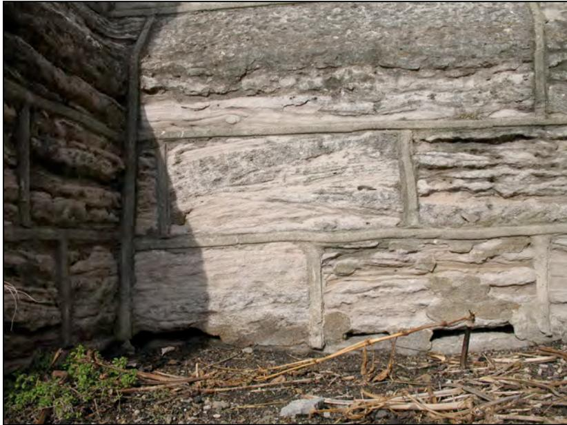
To correct this situation, topsoil should be brought in, spread evenly around the perimeter of the church (using hand tools close to the building), and sloped away using at least a 1:12 pitch to encourage positive drainage. The best time to do this is in the spring or fall, so that the exposed soil can be seeded and then covered with straw.
