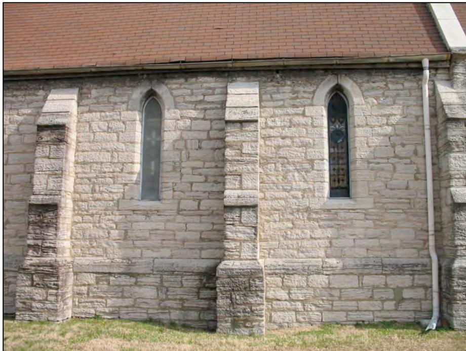
The ends of the leaders are crushed and inhibit proper water flow.
