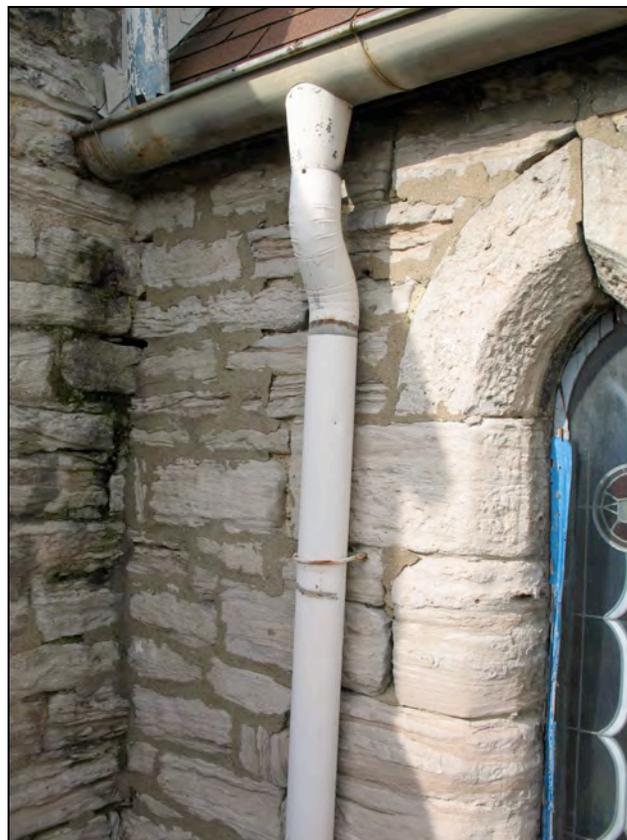
As a result, moss and mold is growing on some of the wall surfaces because of the uncontrolled runoff water.
